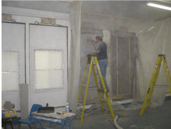
Figure 8. Installation of cellulose insulation in the Charleston Testing Facility.
