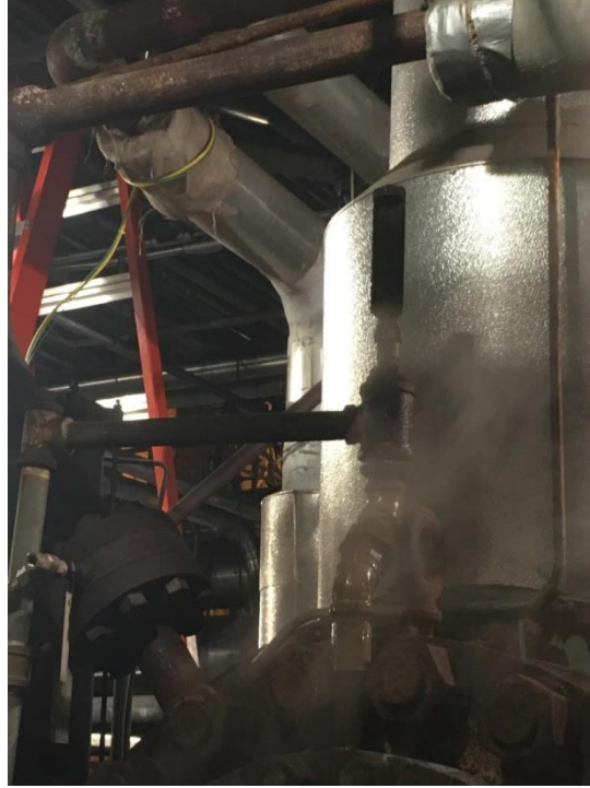
Figure 4. Photograph of test position 2 (boiler feed pump suction).
