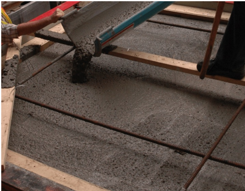
Fig. 1. Use of SCC to allow for consolidation without affecting simulated defects.
