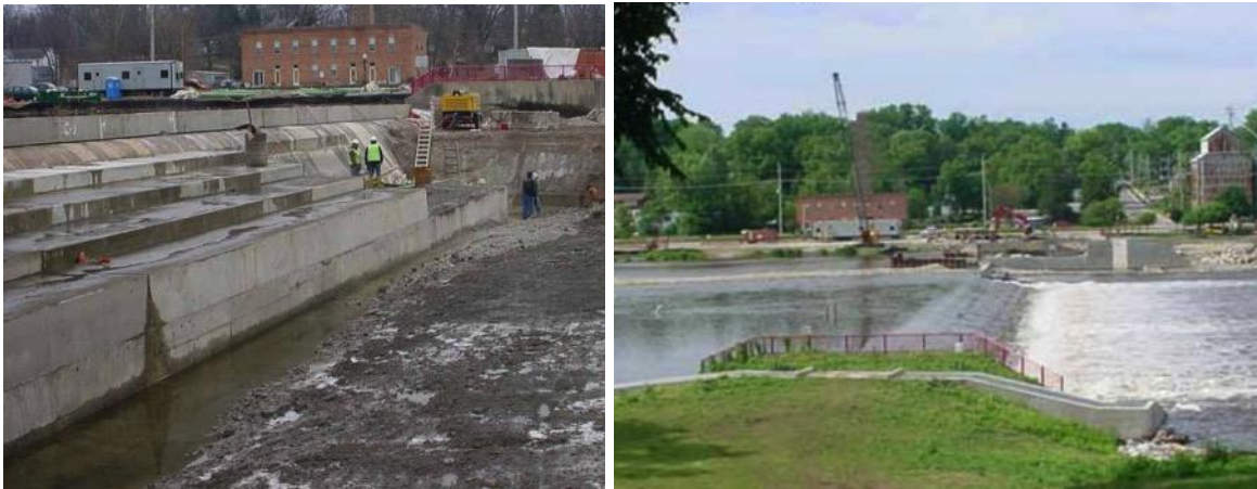
Figure 23. Excavation and construction of a stepped spillway for a low-head dam. (Source: Illinois Department of Natural Resources. Used by permission.)
