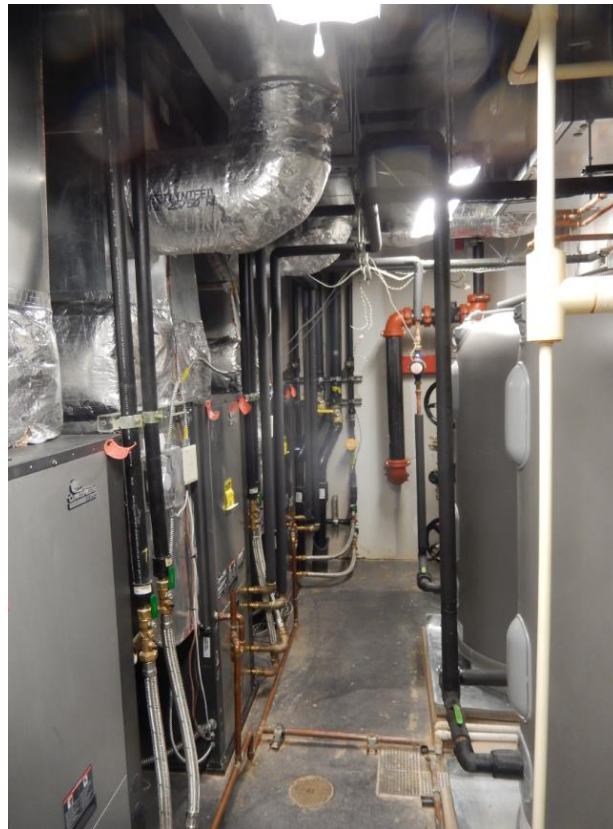
Figure 9. Oklahoma City host building mechanical room; instrumented Trilogy is on rh side against back wall; Trilogy HW tanks at left (Source: ClimateMaster)
