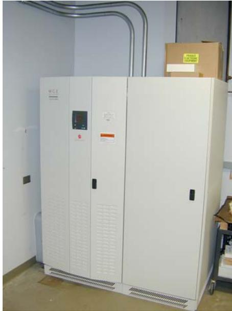
Figure 1. Installed Back-Up Power Supply System for gradient Test Systems
