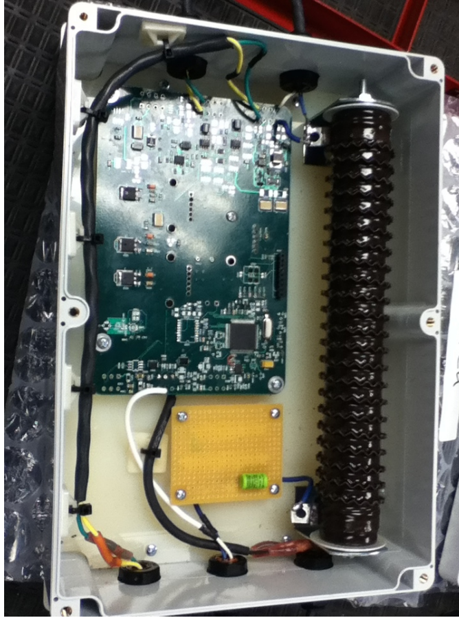
Figure 64. Newly installed T2TCU main circuit board.
