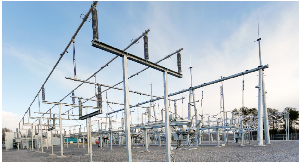
New ORNL electricity substation, completed in FY 2015
