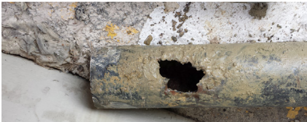
Water saving results from identifying/replacing old water distribution system
