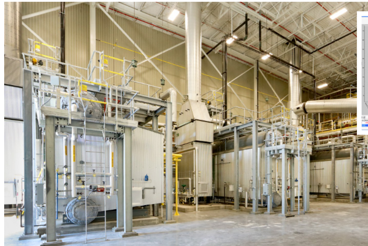
New dual-fuel boilers enhance steam system efficiency
