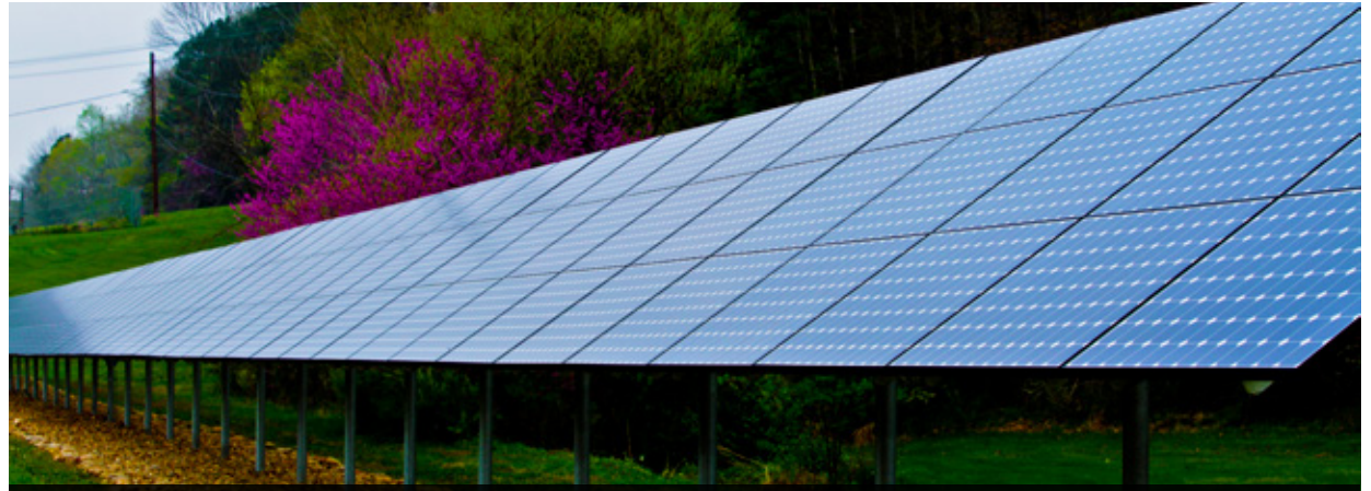
Bethel Valley Road photovoltaic array
