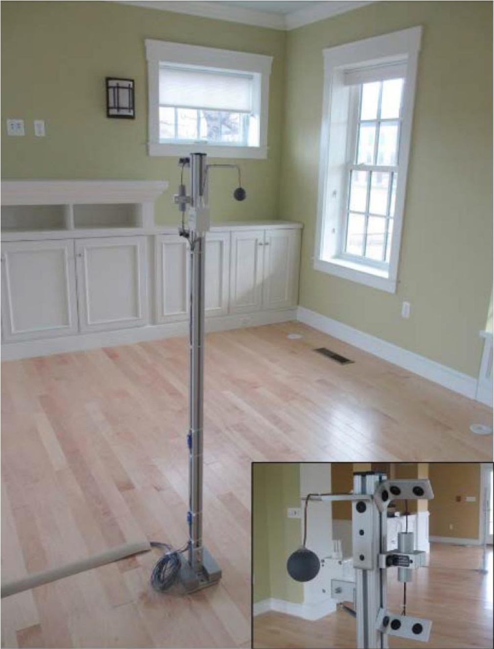
Fig. 4.25. Sensors mounted in center of room to monitor thermal comfort; inset shows closeup of shielded dry bulb temperature sensor, globe temperature sensor, and relative humidity sensor
