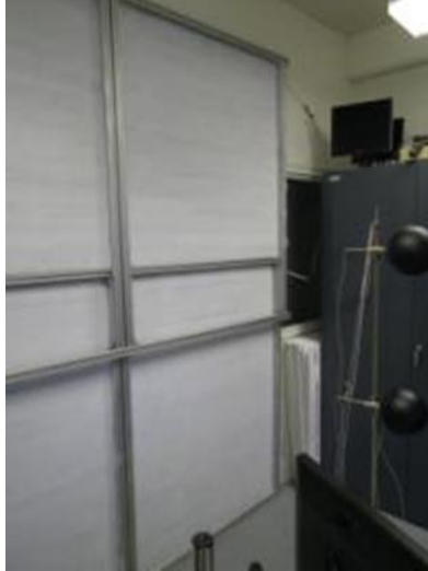
Fig. 2.4. Picture of the radiative HX installed in an office setting
