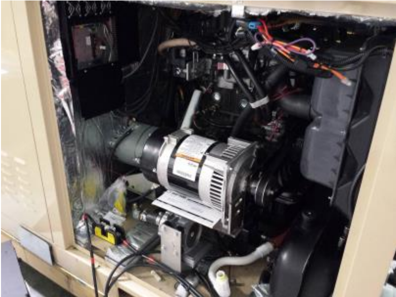
Fig. 3.28. Prototype with low-cost AC generator
