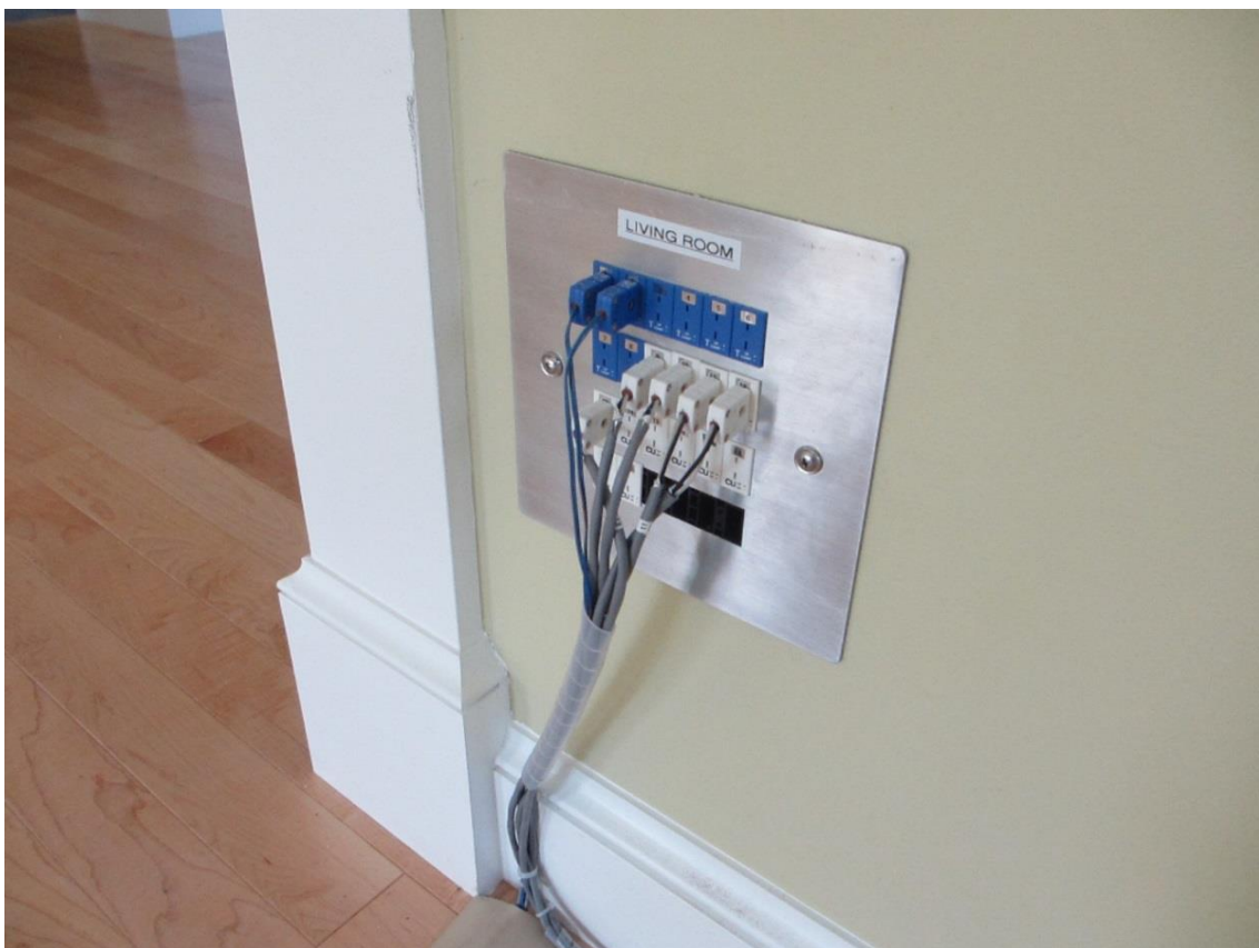
Fig. 4.14. Typical room plug panel
