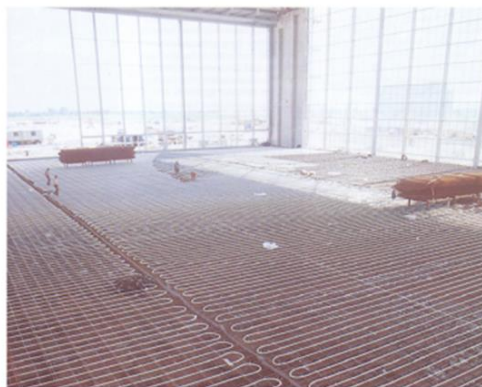
Fig. 2.3. Picture of piping for heated floor system during installation (Olesen, 2011)
