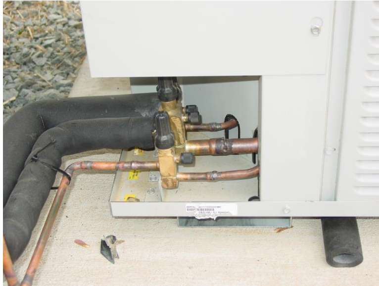
Fig. 4.2. Heat pump indoor unit, refrigerant circuiting/instrumentation (a) and outdoor unit with hot gas reheat piping (b).
