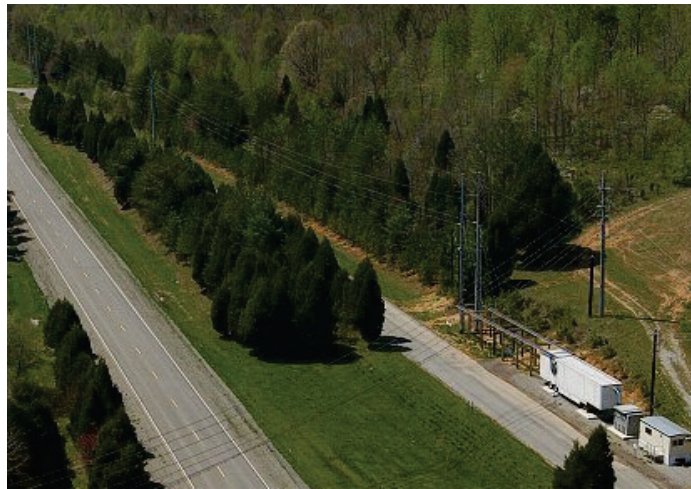
Fig. 5. Aerial view of the Powerline Conductor Accelerated Test facility.
