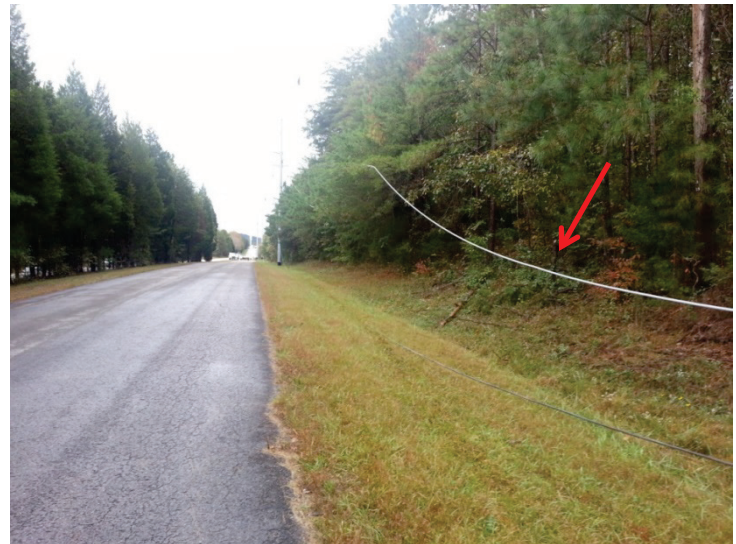
Fig. 12. Payoff reel brake failure caused the Drake/ACSS/MA2/E3X conductor to fall to the ground during installation.
