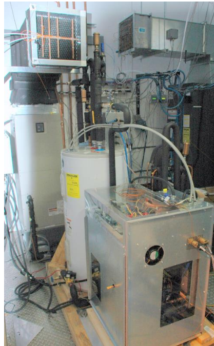
Fig. 9. 2 nd generation AS-IHP lab prototype as set up in ORNL test chamber; compressor/WH package in front, WH tank just behind, and air handler in back (with air flow measurement set up).
