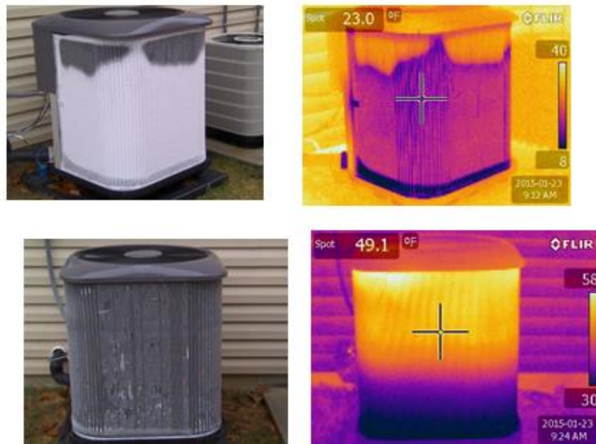
Fig. 21. Frosted coil (top) and after defrosting was completed (bottom).
