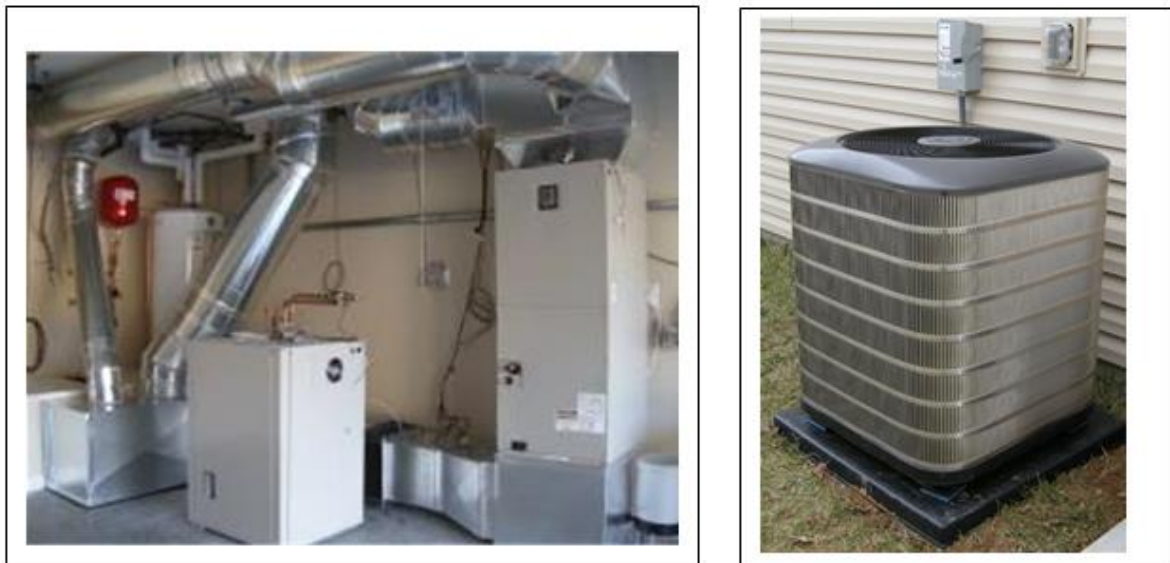
Fig. 13. Field test prototype installation; l) indoor sections (hot water storage tank, compressor and water heating module, and indoor fan coil), r) outdoor fan coil section
