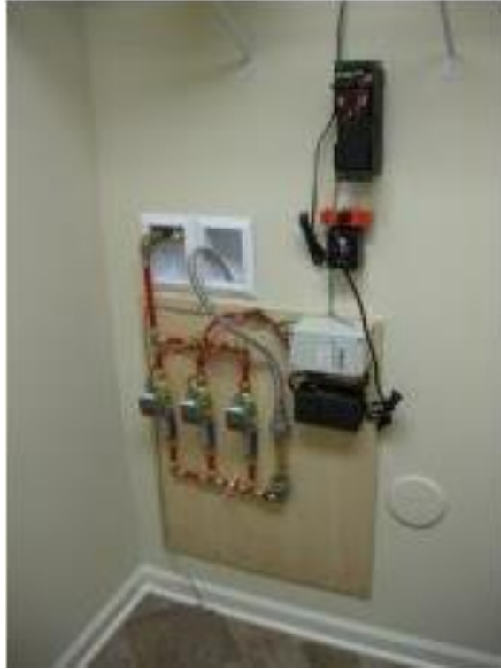
Fig. 15. Hot water use control valves
