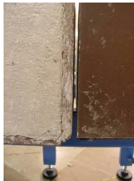
Fig. 1-44. Gap between scattering box concrete blocks.
