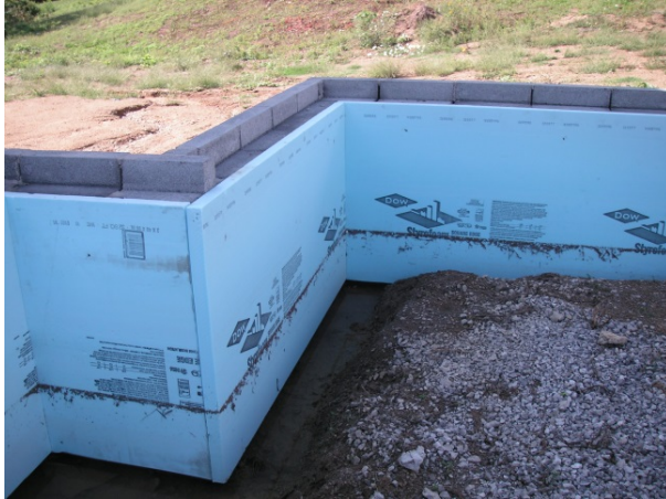
Interior foundation wall insulated with 2 in. XPS
