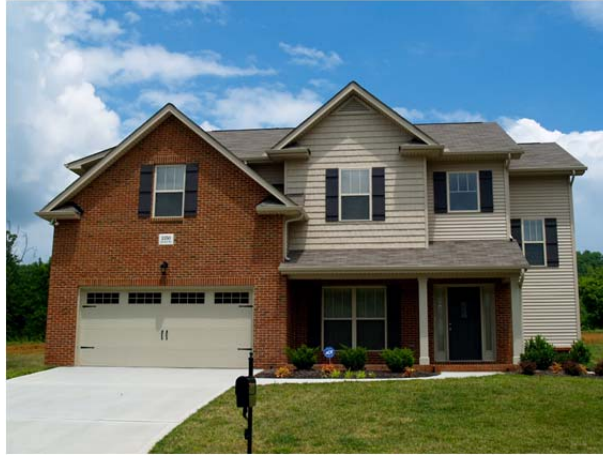
Fig. 11. Front view of the retrofit (CC2) home as viewed from the Hillman Rd.
