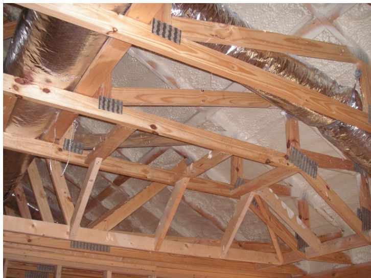
Fig. 14. CC2 sheathing with 1 in. of ccSPF insulation.
