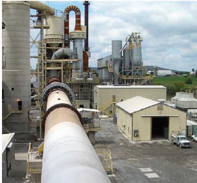
Figure 11. WHP from Lime Production
