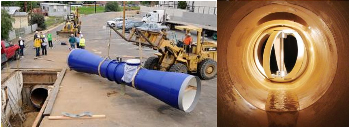
Fig. 6.6. Installation of a Lucid Pipe system (left) and internal view of runner (right). (Source: Lucid Energy Systems)
