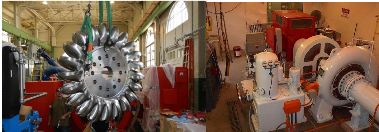
Fig. 6.3. Installation of a new runner in the modernization of the Boulder Canyon plant (left) and treated water moving through the system at the Sunshine hydro plant (right). (Source: City of Boulder, Colorado)
