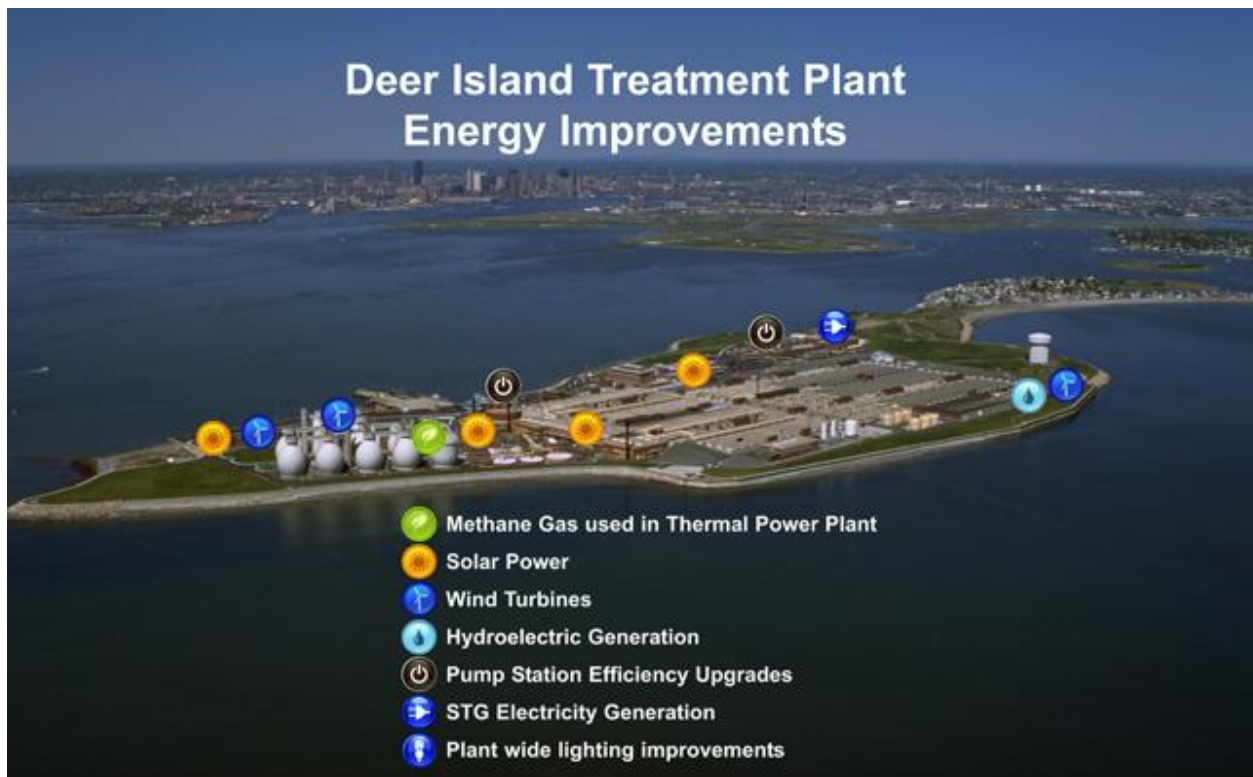
Fig. 6.2. Photograph of energy improvements made on Deer Island. Includes conduit hydropower that was added to the treatment plant outfall; STG = “steam to gas.” (Source: MWRA)
