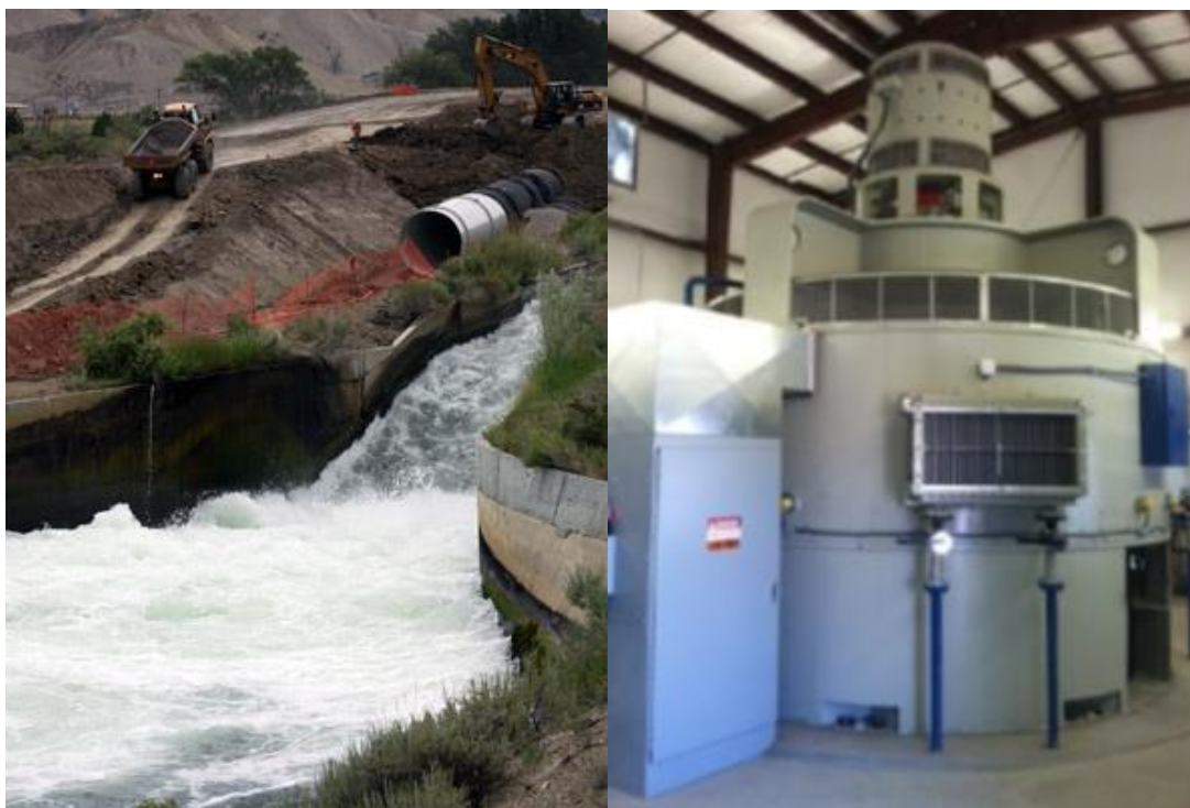
Fig. 6.1. Photographs of the South Canal Project. (Source: DMEA)
