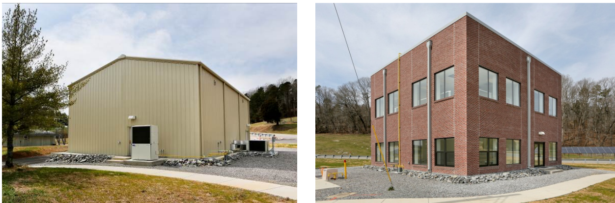
Figure 2. Flexible Research Platforms cladded to emulate 1980s metal buildings (left) and office buildings from the 10-county Greater Philadelphia region (right).
