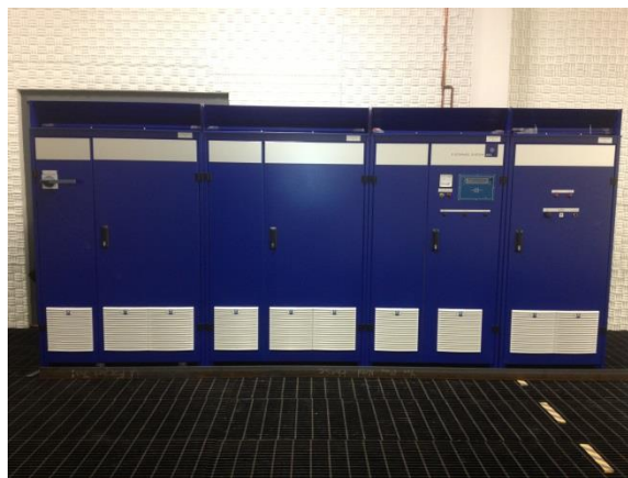
Figure 2: AVL e-storage unit installed at ORNL VSI laboratory.
