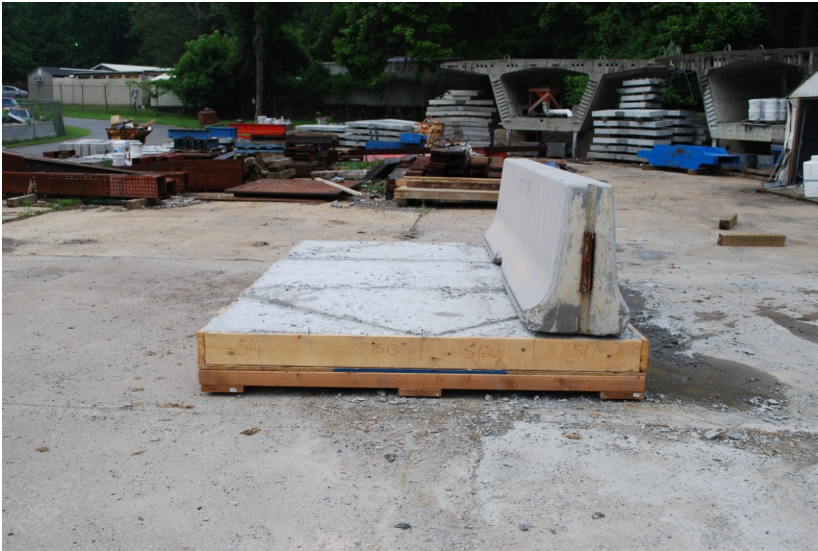
Figure 20. Concrete barrier anchored to mockup bridge deck slab.
