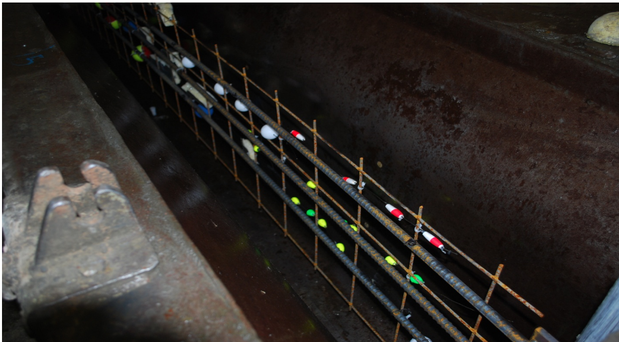
Figure 15. F-shaped free standing portable barrier fabrication.
