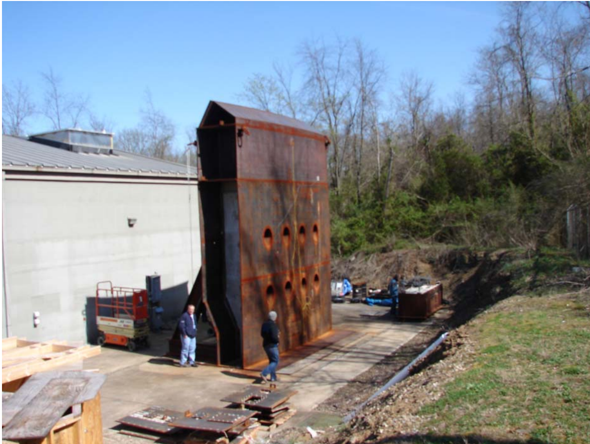
Figure 7. WesDyne Westinghouse AP1000 Shield Building NDE Evaluation Section.
