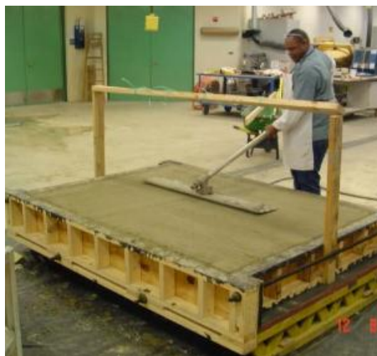
Figure 44. Finishing concrete surface
