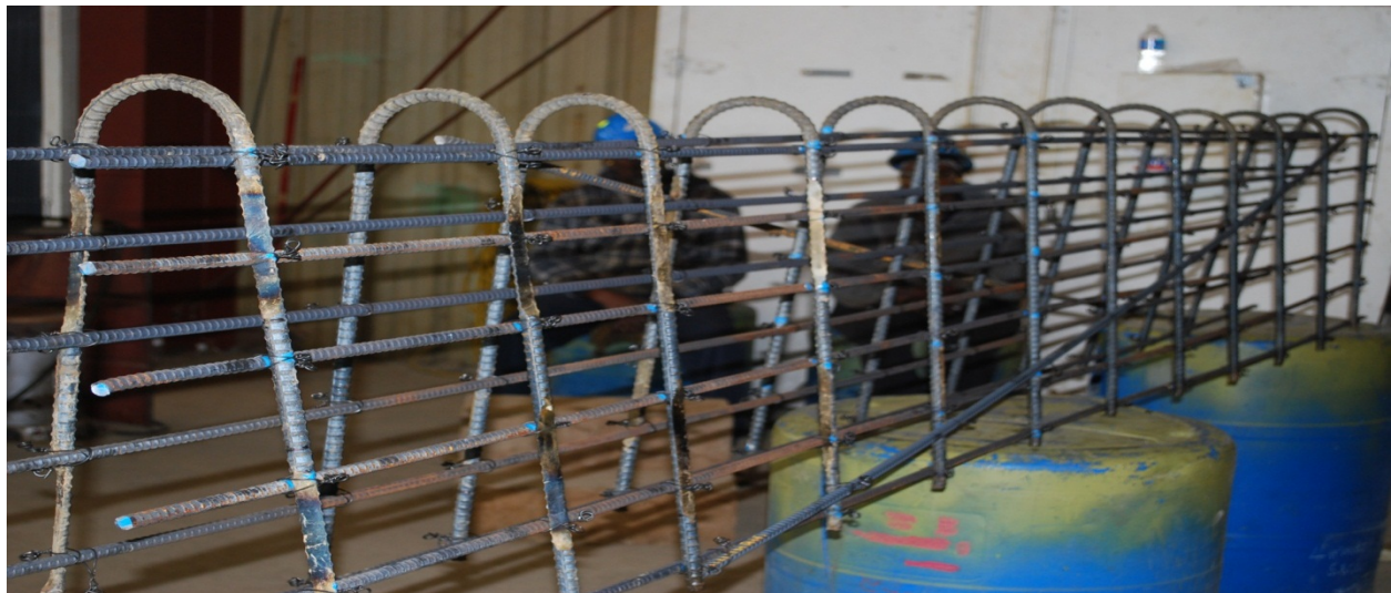
Figure 13. F-shaped bolt-down barrier fabrication with simulated corrosion.
