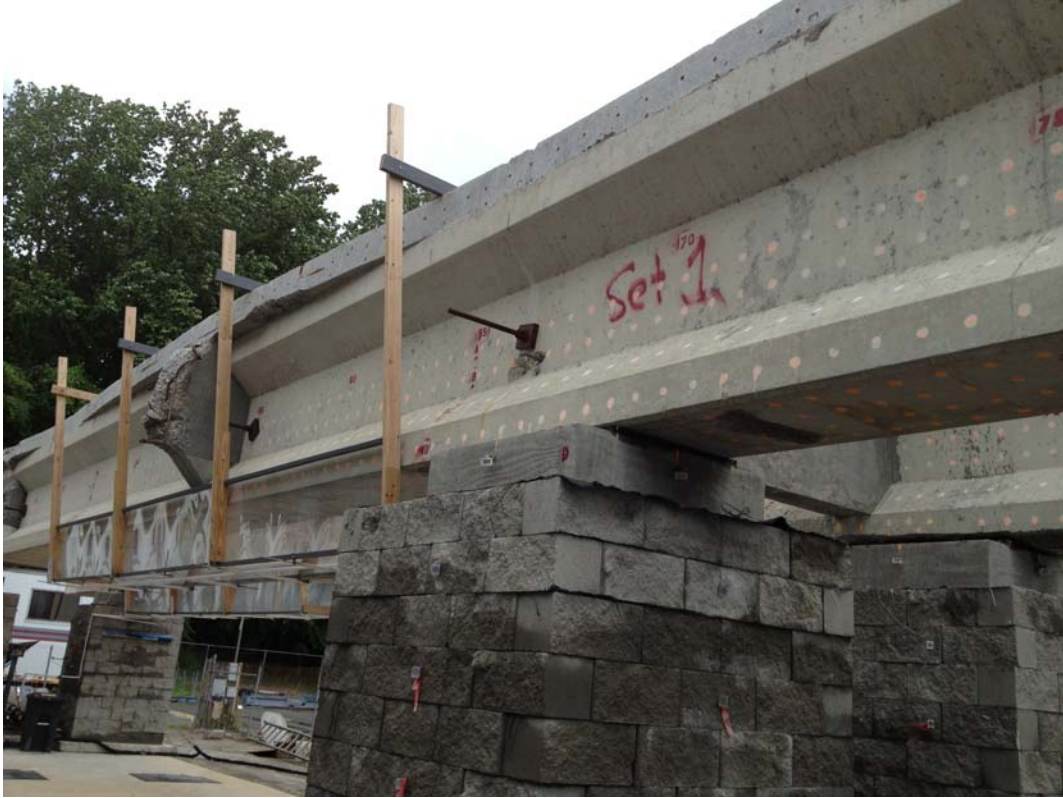
Figure 27. Bridge support specimen undergoing steel reinforcement corrosion testing.
