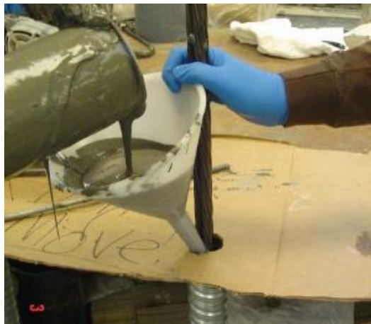
Figure 40. Filling duct portion entirely full
