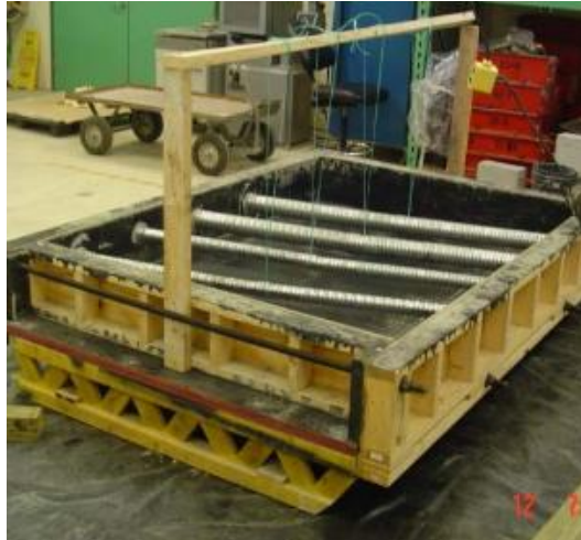
Figure 42. Ducts placed in framework
