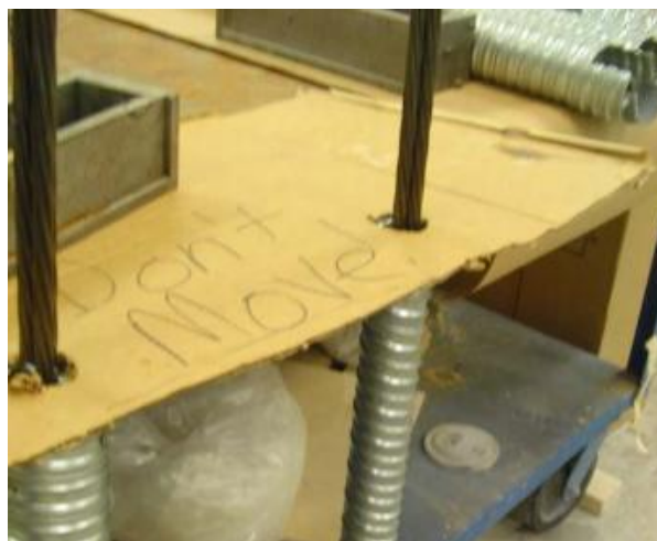
Figure 41. Fully filled duct sections curing
