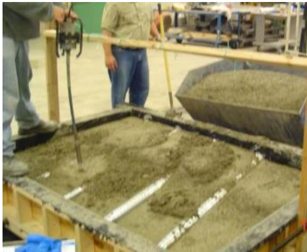
Figure 43. Pouring and compacting concrete
