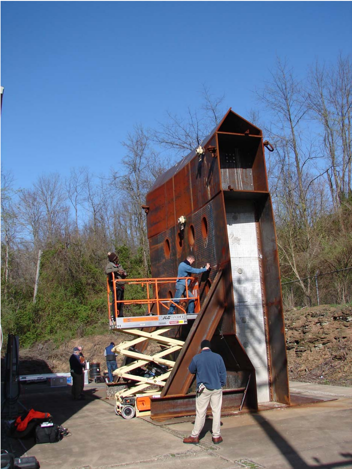
Figure 8. NDE Evaluations being performed on AP1000 Shield Building Section.
