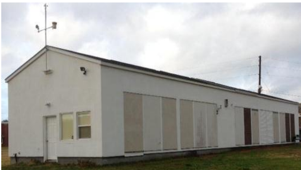
Figure 1. Charleston, SC NET facility.
