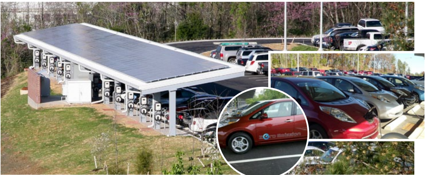
ORNL solar-assisted charging station
