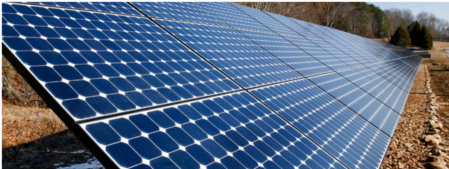
Bethel Valley Road 51.25kW Solar Array
