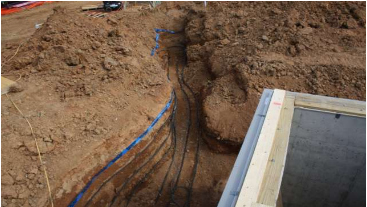
Figure 2.9. HGFX installed in a utility trench.
