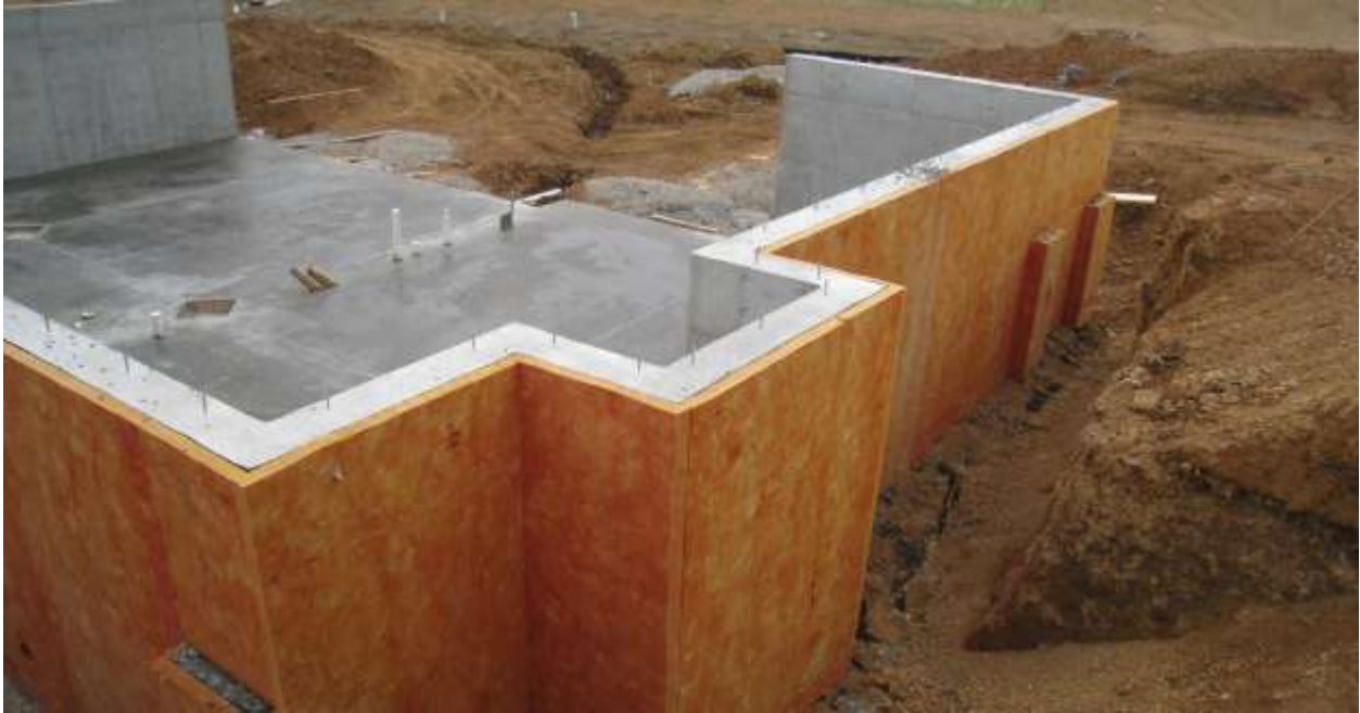
Figure 2.6. FHX/HGX supply and return headers (brown covering) installed up through basement floor.
