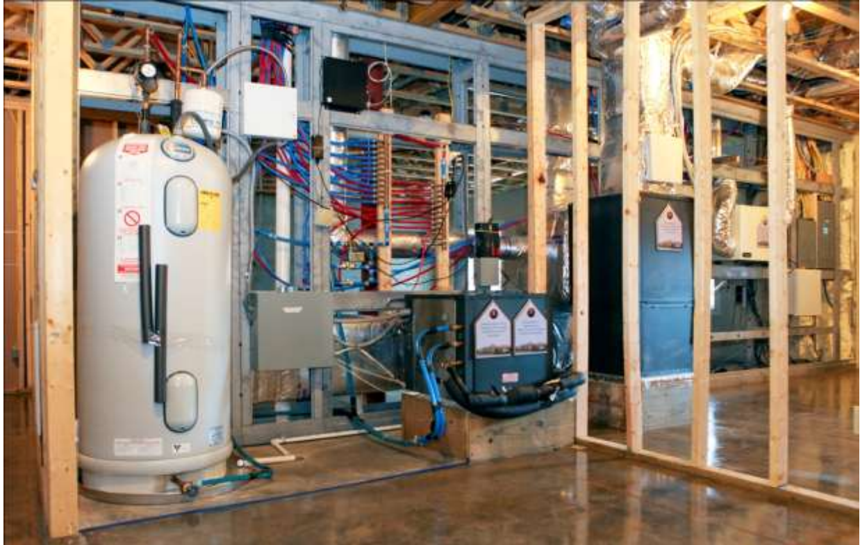
Figure 2.3. Space conditioning equipment (WAHP on right) and water heating equipment (WWHP and associated tank on left) at House 1.
