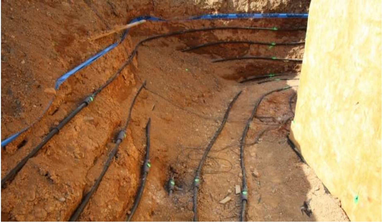
Figure 2.8. FHX installed in overcut around a basement wall exterior corner.
