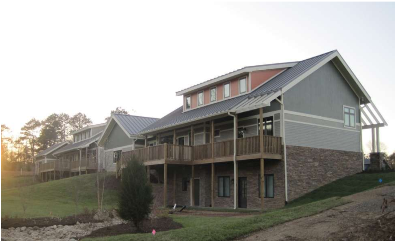
Figure 2.2. Rear view of House 1 (left) and House 2 (right) showing the walkout basements.
