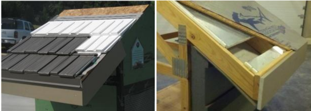
Figure 25. Prototype assemblies of WC3 roof (left) and WC4 roof (right).
