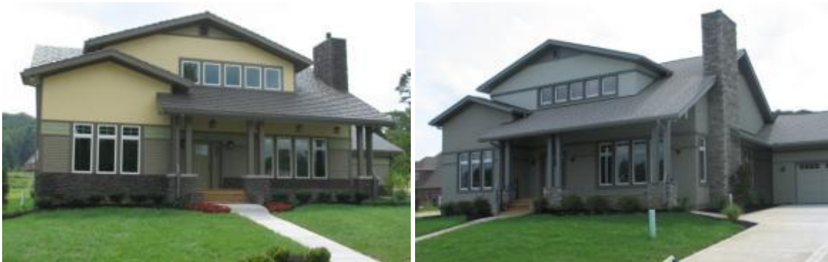
Figure 26. Exterior painting and cladding for WC3 (left) and WC4 (right)
