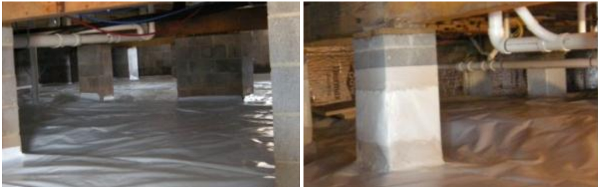
Figure 30. Vented crawlspace in WC3 (left) and walls insulated and sealed in WC4 crawlspace (right)
