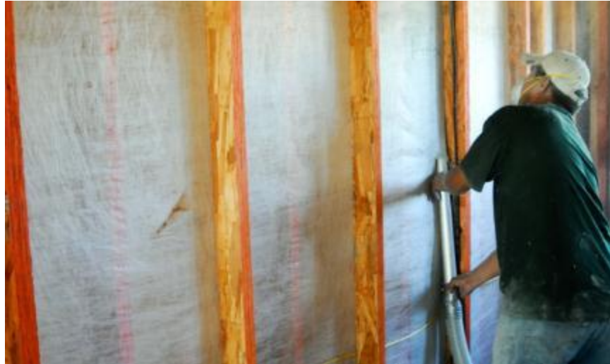
Figure 28. Insulation addition in the double-stud wall assembly of WC3
