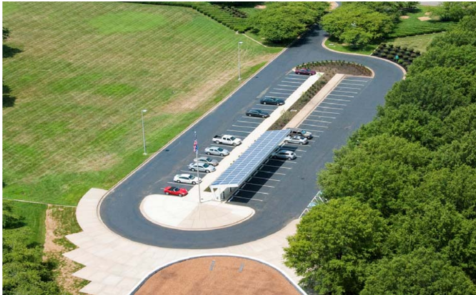
Nissan Smyrna Administration Building Solar Canopy
