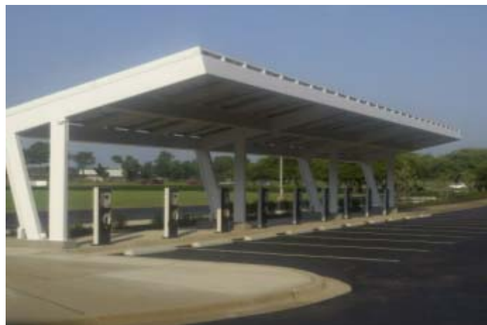
Nissan Smyrna Administration Building EVSEs
