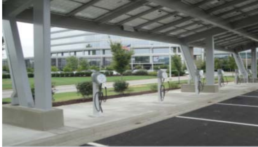
Franklin, Nissan Headquarters EVSEs
