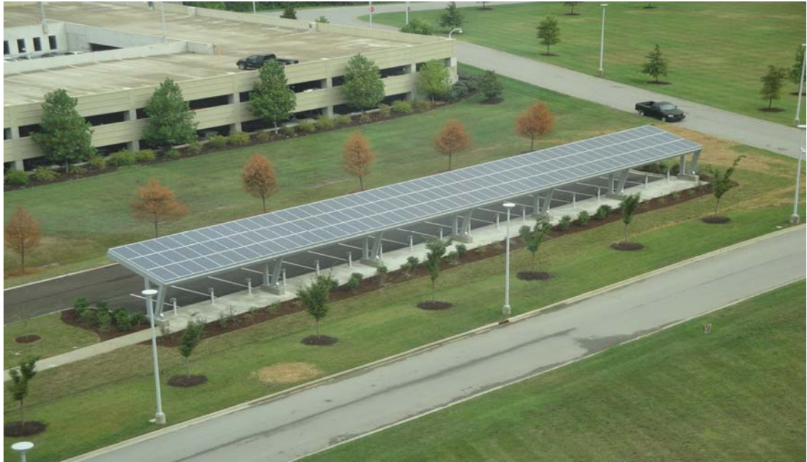
Franklin, Nissan Headquarters Solar Canopy
