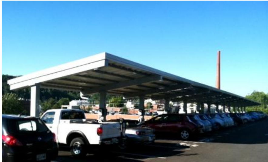
ORNL Solar-Assisted EV Charging Station
