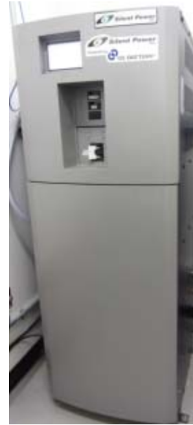
EPRI Silent Power Battery System
