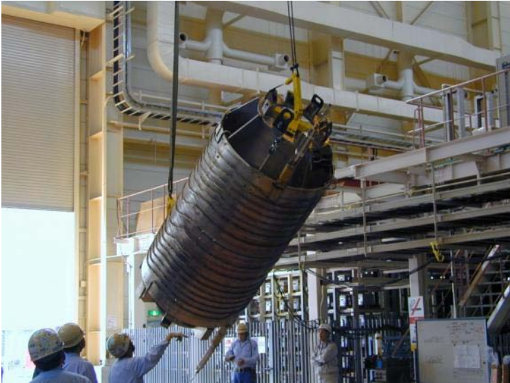
Fig. 14. TF Insert Coil turnover procedure during installation into a center hole of the CSMC.
