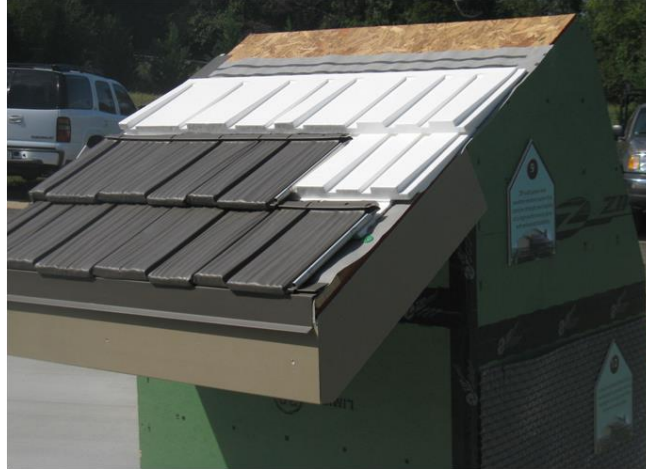
Figure 1. Prototype assembly of WC3 roof.
