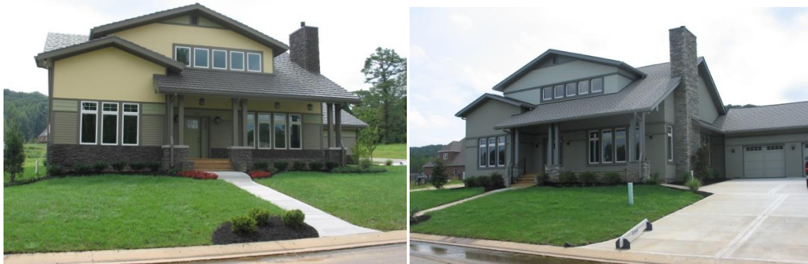
Figure 3. Exterior painting and cladding for WC3 (left) and WC4 (right)
