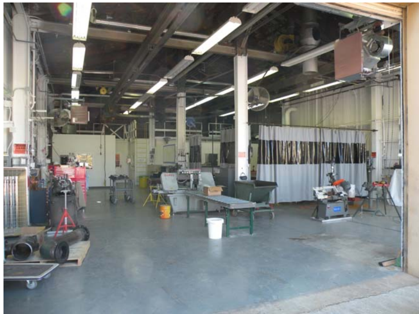
Fig. 4. Refurbished Oak Ridge National Laboratory pipe shop.
