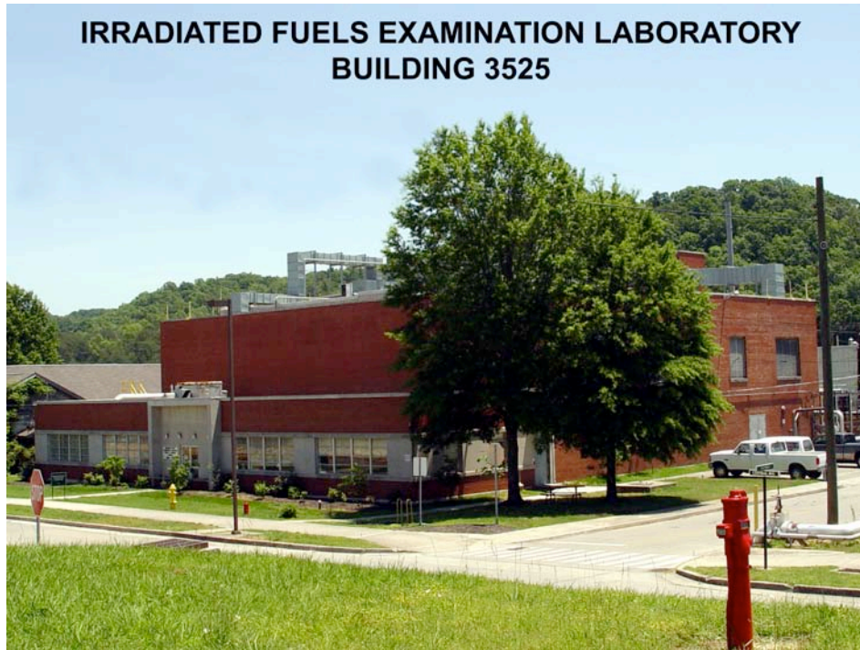
Fig. 1. Building 3525 at ORNL
