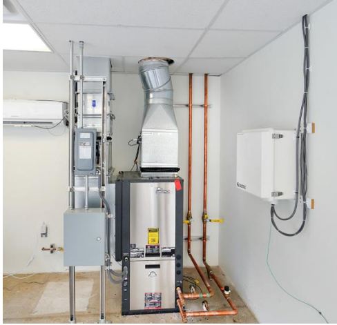
State-of-the-art 2-stage GSHP
