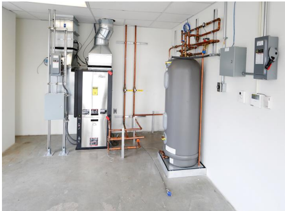
Integrated GSHP with hot water generation
