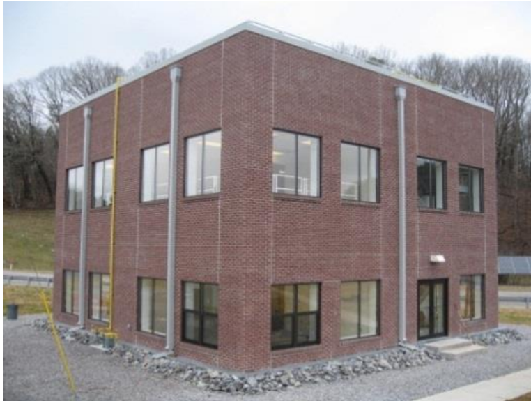
Figure 1. The building hosting the flexible DGSHP system test facility.
