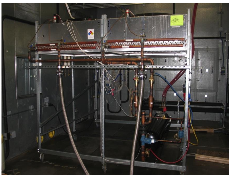
Fig. 23. Air-cooled condenser (top) mounted above liquid receiver (bottom).
