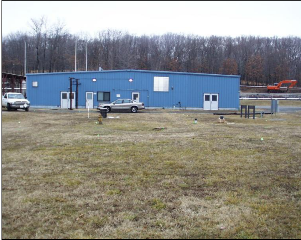
Figure 4.2. Location of the Raman Sensor Field Demonstration at the IHDIV Site.
