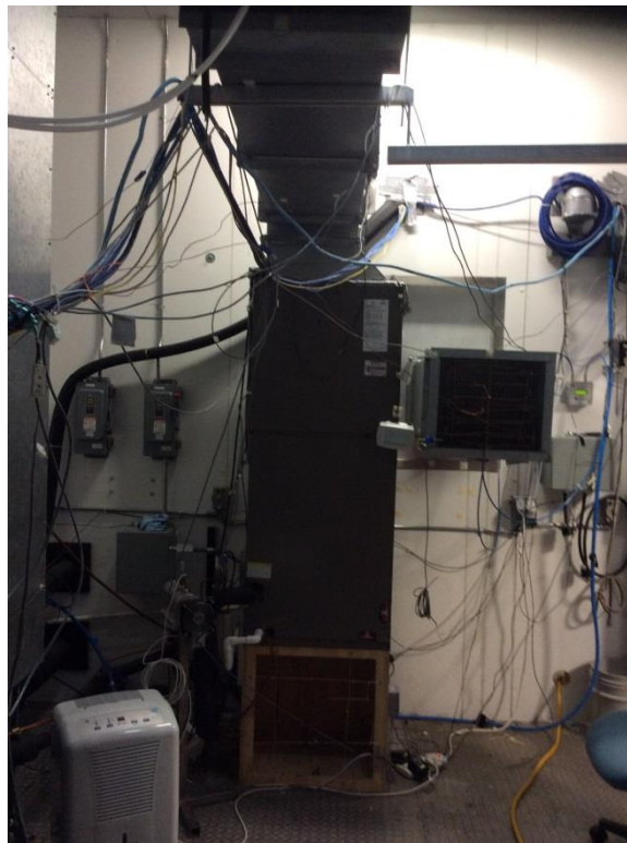
Figure 47: Lab Prototype – Indoor Air Handler
