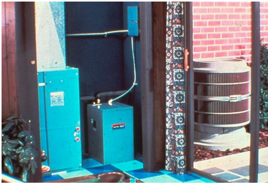
Figure 11: Early 1980's 3-piece ASHP design for northern climate applications
