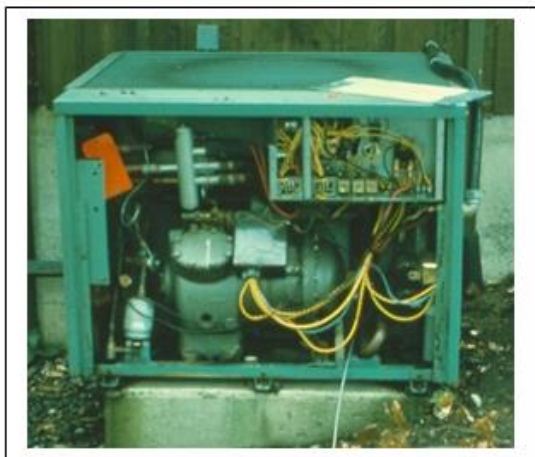
Figure 6: Sample outdoor sections of heat pumps field tested from 1976-1978: left, ca 1960's unit installed in Seattle residence (note semi hermetic compressor); right, ca 1970's unit originally installed in Minneapolis residence (note - unit was undersized)
