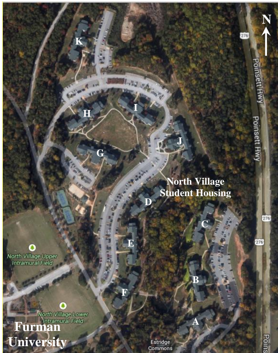
Fig. 1. Aerial view of the GSHP demonstration site at North Village student housing at Furman University.
