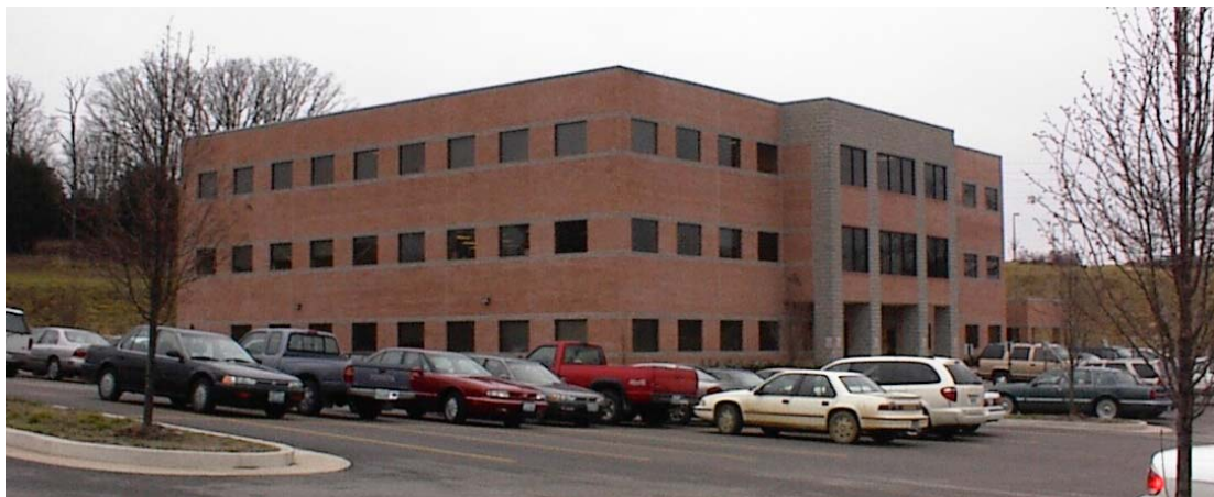
Fig. 11. The Jefferson City office building that was evaluated.
