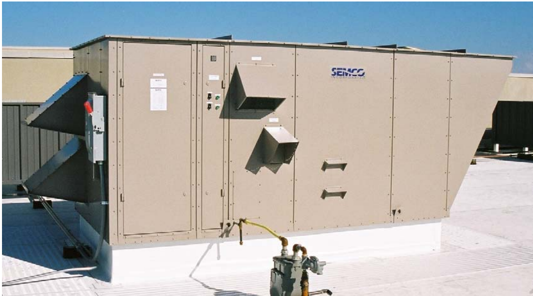
Fig. 13. SEMCO IADR system installed at a pilot site location.
