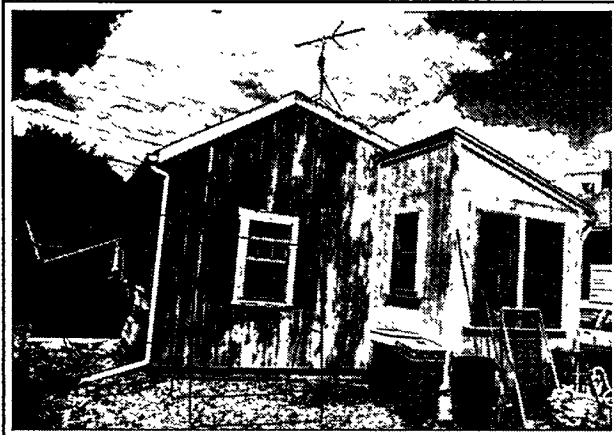
The interface between old and new is often a trouble spot.
