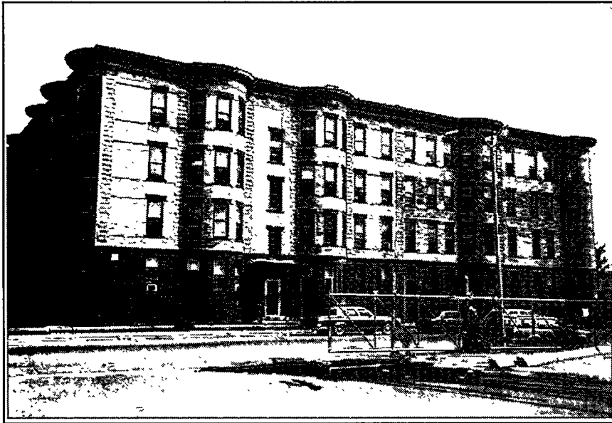
This is a large multifamily dwelling in Holyoke, Massachusetts, which was weatherized by HAP Inc., from Springfield, Massachusetts.
