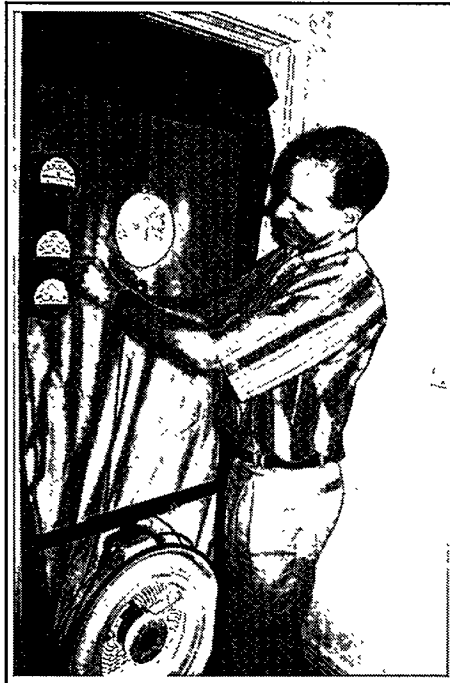
Blower door setup, inside view. The technician is zeroing the gauges, so as to measure both air flow and the inside-outside pressure difference caused by the blower door. The speed of the fan is adjusted using the control on top of the fan.
