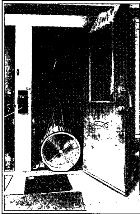
Blower door setup, outside view.
