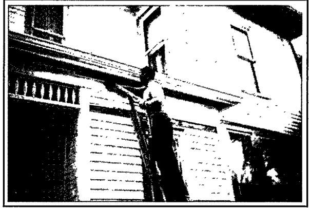
As revealed by a blower door and a pressure gauge in a test that takes only several minutes, the area under this porch is directly connected to the envelope through floor joists between the first and second floor. High-density insulation is being used to air-seal this largest hole in the dwelling.
