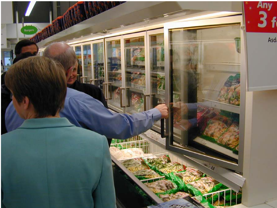
Figure 16 - Example of freezer case type tested by UK team in environmental chamber to determine impact of store temperature, relative humidity and ventilation mode (conventional or displacement) on performance
