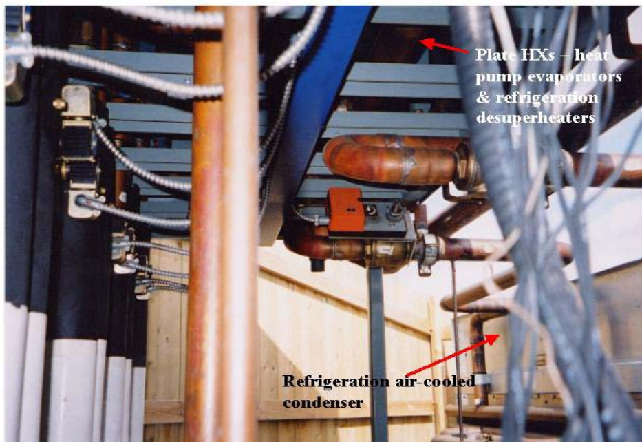
Figure 10 – Plate heat exchangers (HX) for heat pump evaporators and refrigeration desuperheaters and subcooler
