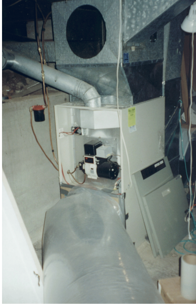
Fig. 2.2. The Aeroseal tubing connection.
