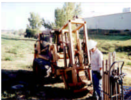
U.S. DoD and DOE representatives conduct a joint evaluation of the hydraulic performance of PRBs at former Lowry Air Force Base
