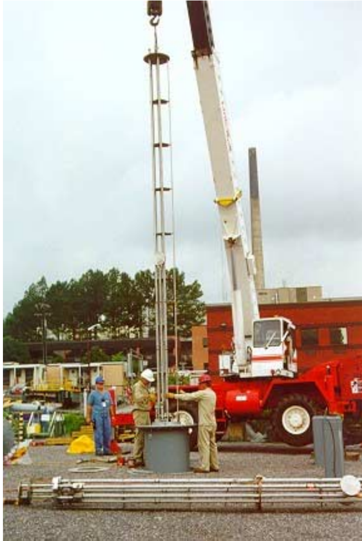
Fig. 2. PulsAir Mixer during installation at GAAT W-9.
