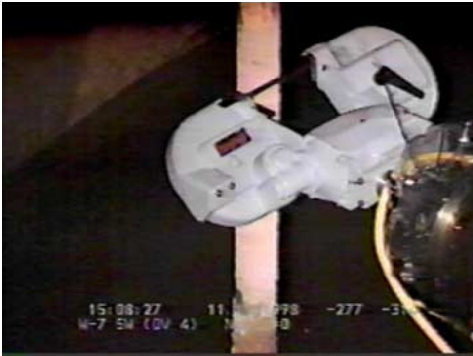
Fig. 7. Pipe-cutting tool in use in GAAT W-7.
