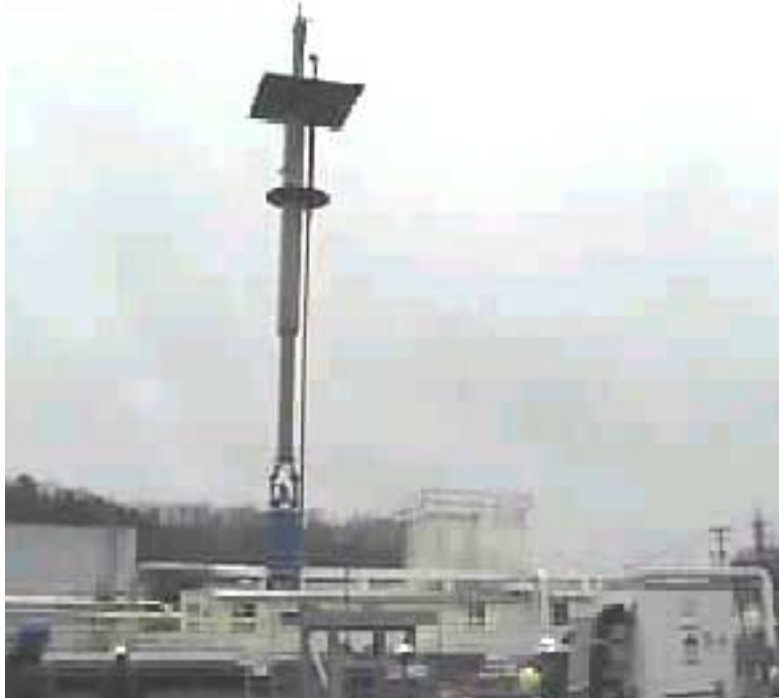
Fig. 8. Installation of the WTP in GAAT waste consolidation tank W-9.
