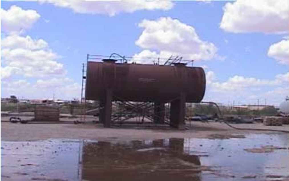
Fig. 2. Photograph showing a general overview of the test tank used during the FY 1999 cold demonstration of MPI technology.
