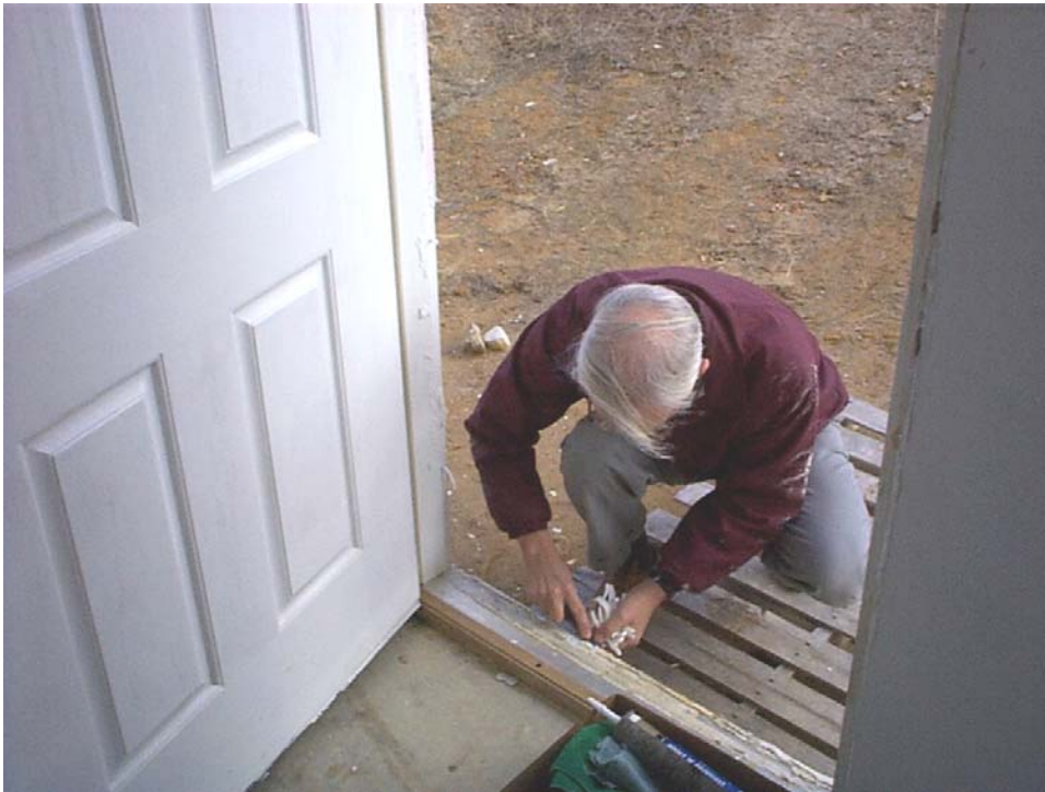
Figure 6-28 Silicon II caulking was installed on the threshold. Prior to reinstalling the polystyrene foam flood dams
