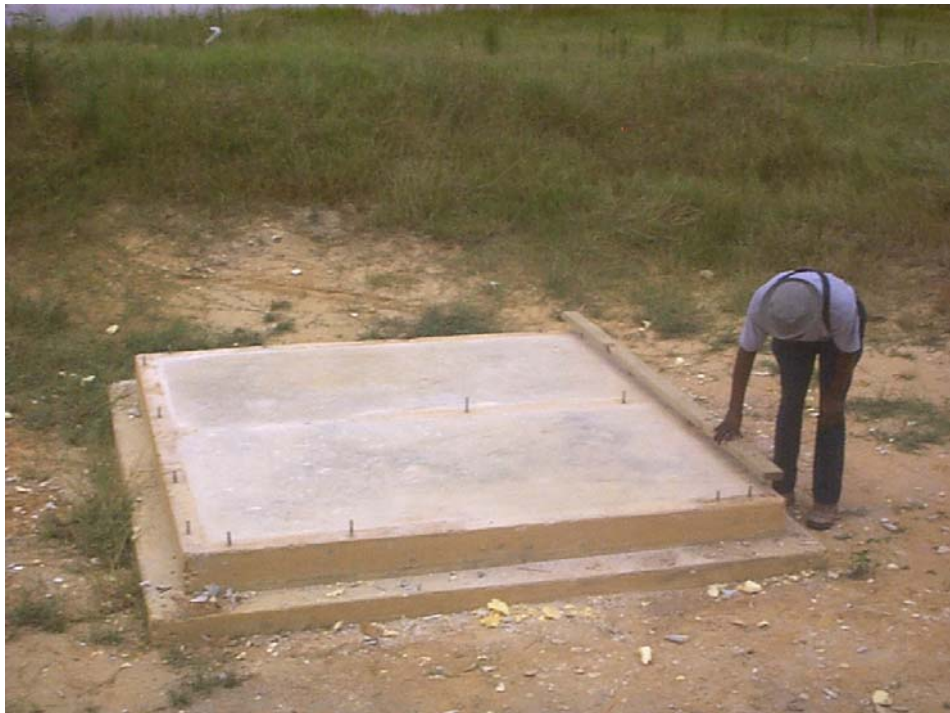
Figure 5-19 Module S-2 - Foundation of module at demolition
