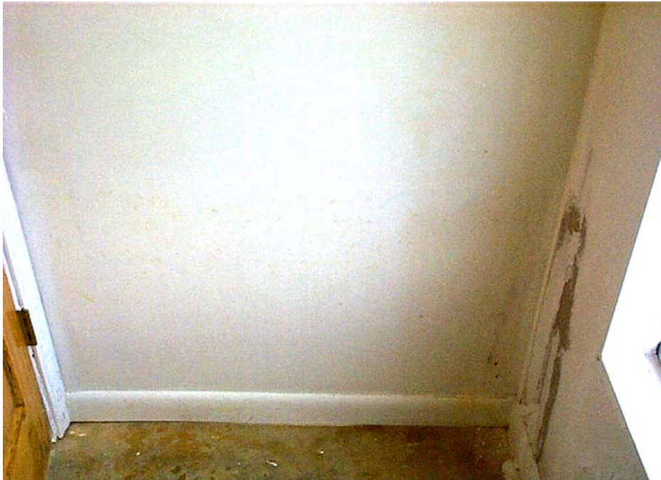
Figure 5-7 Module S-2 (Wall 4) Day 15 - After sanitizing. Mold discoloration gone, some staining remains
