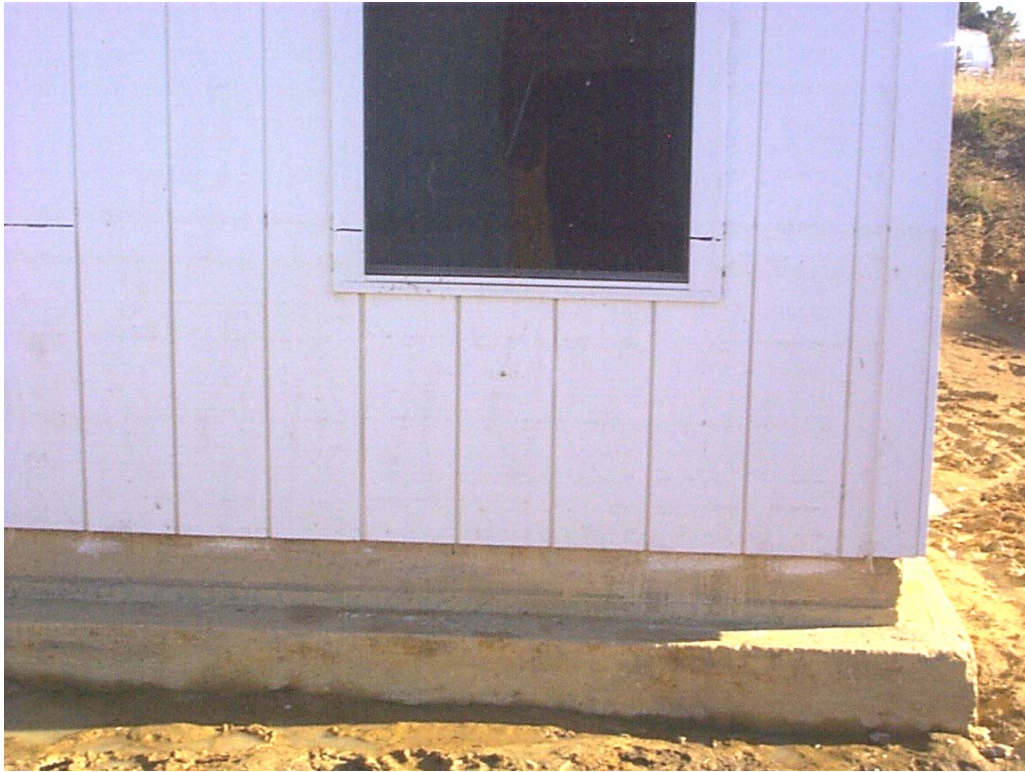
Figure 4-15 Module S-1 (Wall 1, North Exterior Wall) Post-flood, Day 8 (before washing). Walls are stained below flood level.
