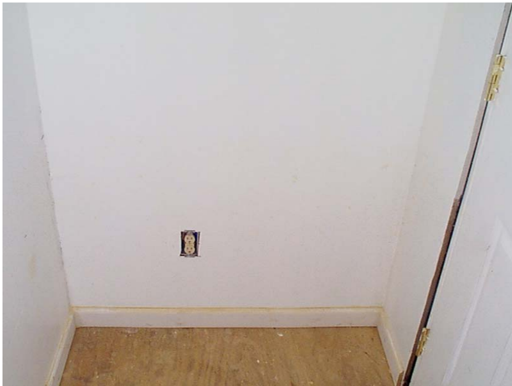
Figure 6-14 Module C-3 (Wall 2) Day 15. No sanitization occurred and no mold growth appeared; wall is restorable.
