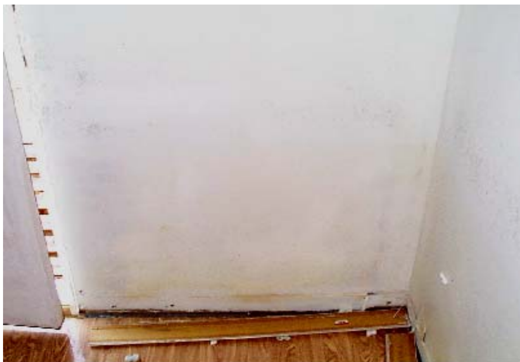
Figure 6-8 Module S-3 (Wall 3) Day 8 – Before washing. Wall is stained and there is mold growth.
