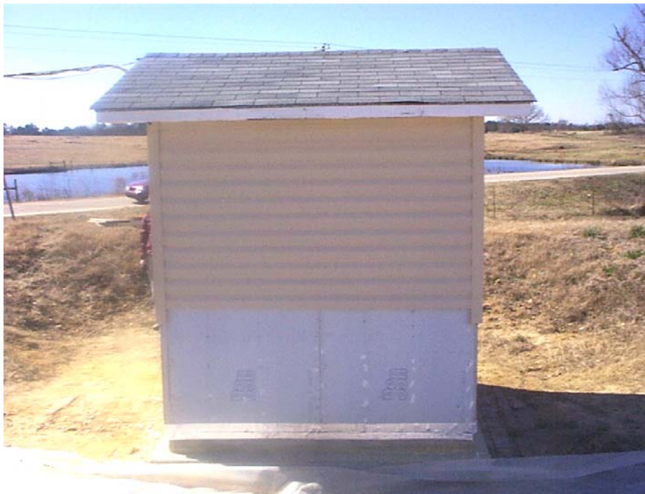
Figure 6-32 Module S-3a, east wall with adhesive sealant tape installed. Prior to flooding
