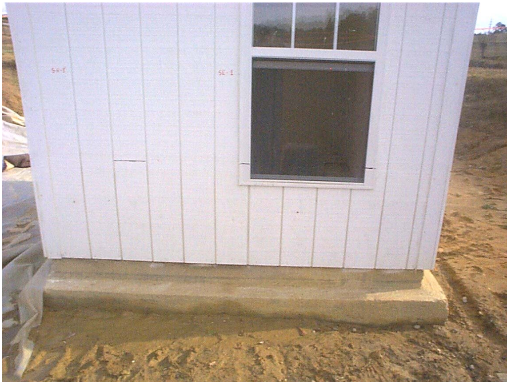
Figure 4-16 Module S-1 (Wall 1, North Exterior Wall) Post-flood, Day 15 (after washing). Wall remains slightly stained.
