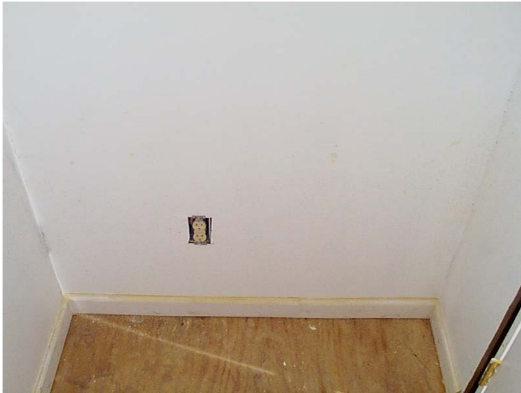
Figure 6-13 Module C-3 (Wall 2) Day 10 - After washing with water. No visible mold stains.
