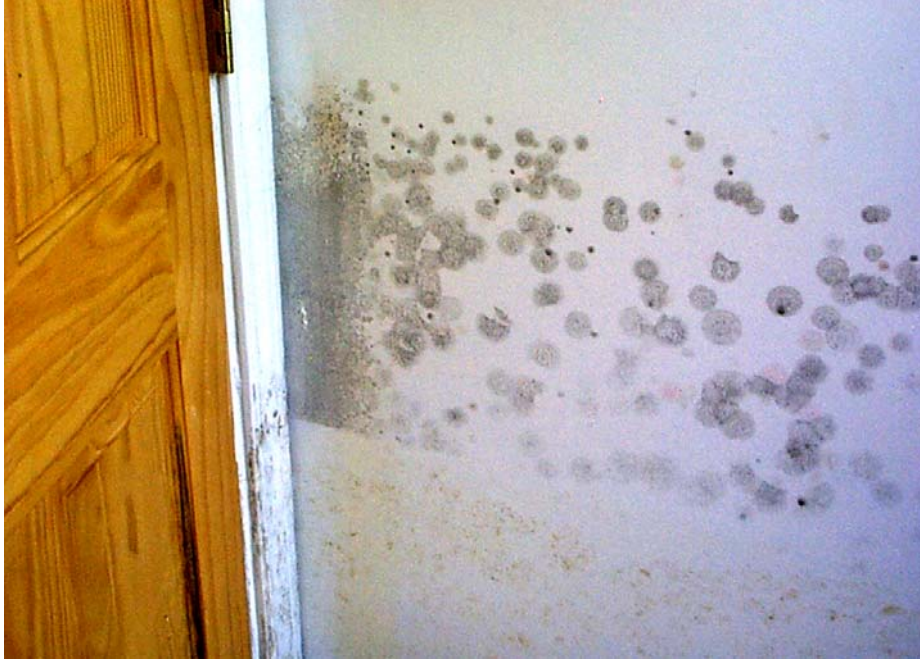
Figure 5-6 Module S-2 (Wall 4) Day 10 - After washing with water. Mold growth and staining on walls
