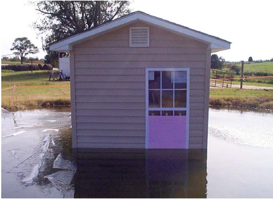
Figure 6-2 Module S-3 Wall 1. Dam on window during flooding is staying in place.
