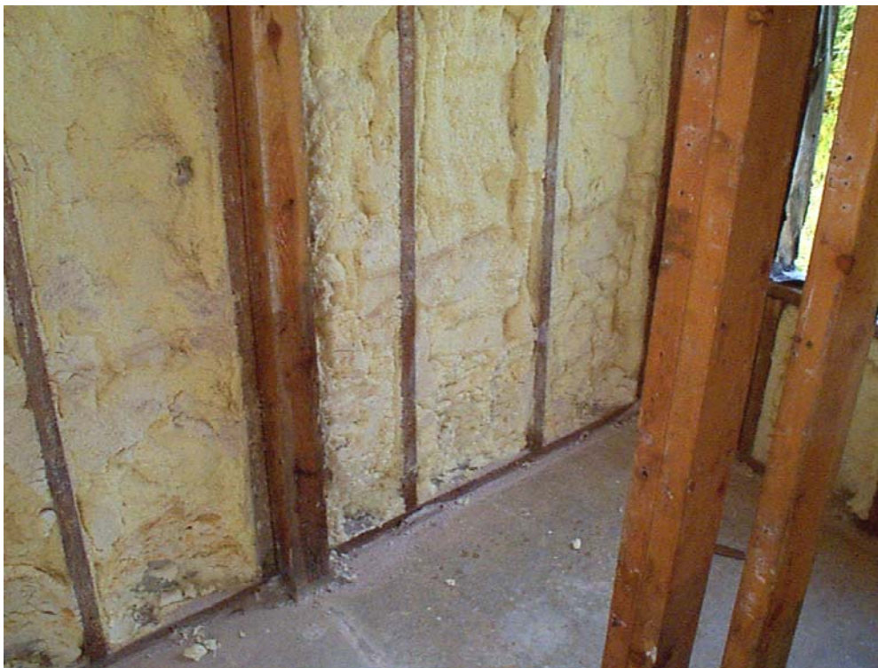
Figure 6-17 Inside of Module S-2 (Wall 4) at autopsy. Insulation and wall cavities are dry and in good condition
