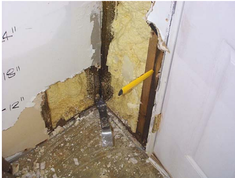
Figure 6-35 Module S-3a Interior southeast corner of Room S-301 after second dry flood proof test. Water entered the module during flooding through the crack between the doubled studs (yellow knife) that form the door rough framing. It also entered through the crack between the corner studs and the sill plate (grey pry bar).
