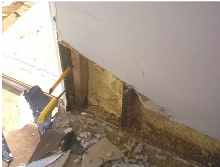
Figure 6-36 Module S-3a Interior south wall after second dry flood proof test. Water entered the module during flooding through the crack between the doubled studs (yellow knife and saw) that form the door rough framing.
