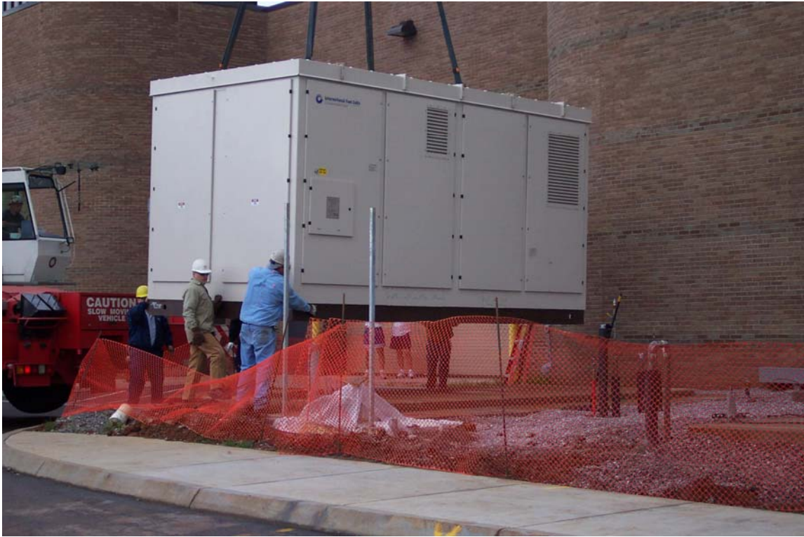
Figure 8. Fuel Cell Being Unloaded
