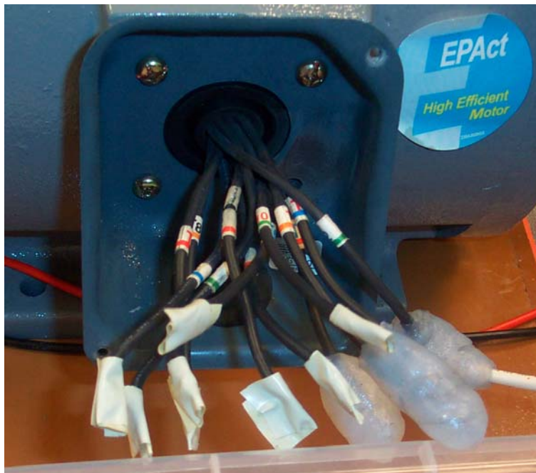
Fig. 10. Two (2) phase leads floating for a phase-to-ground test of a mush-wound stator.
