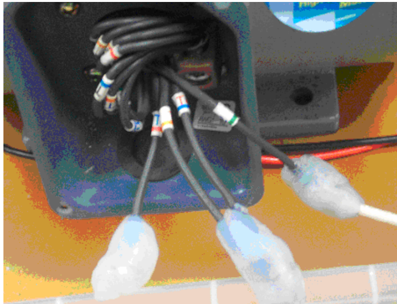
Fig. 8. Phase leads connected to ground for a combined phase-to-phase and phase-to-ground test.
