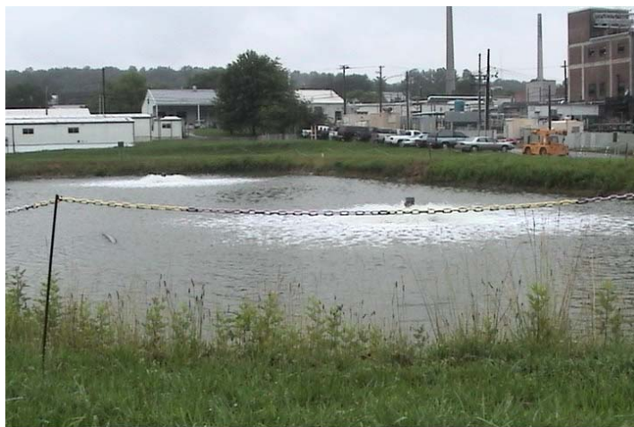
Figure 5-4. One of two sewage treatment lagoons located south of White Oak Avenue.
