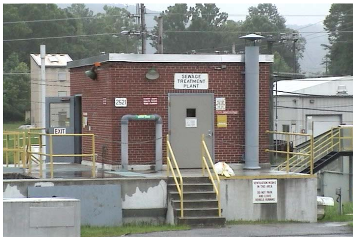
Figure 5-3. The Sewage Treatment Plant (STP), is located in Building 2521 just east of First Street and south of the sewage treatment lagoons.
