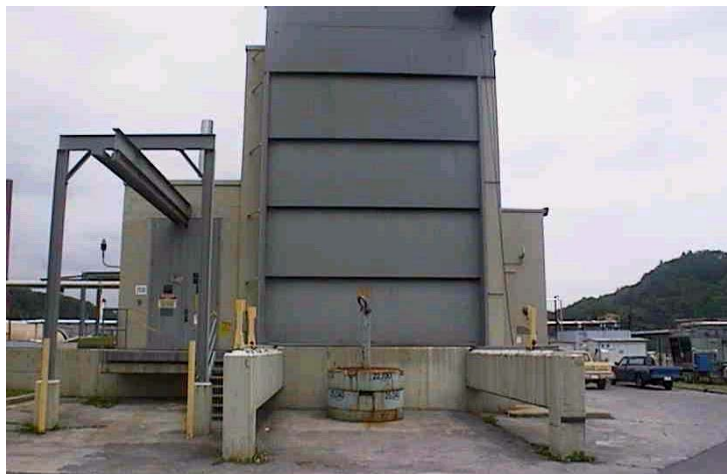
Figure 5-7. Building 2531 is the LLLW Evaporator Facility, which contains 2 evaporators for LLLW.
