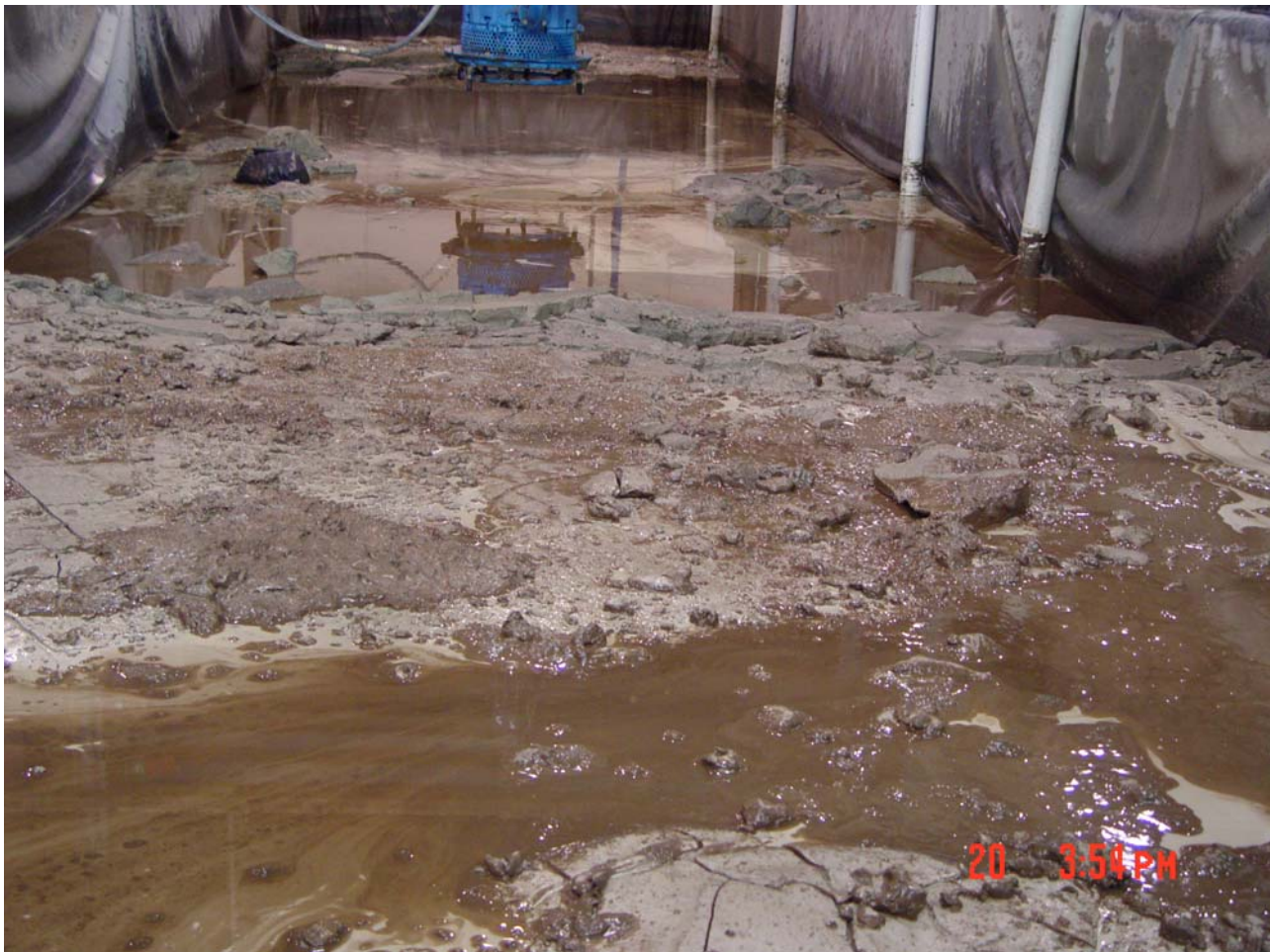
Fig. A.8. Surrogate tank covered with BentogROUT after to Run ITL-4.
