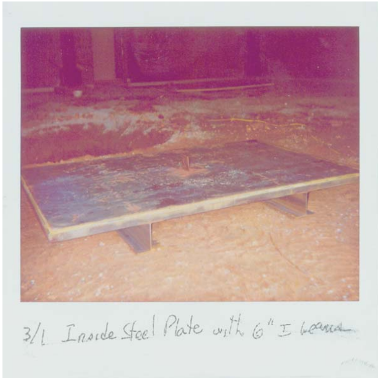
Fig. 11. Interior drop pad steel plate with 6" I-beams.
