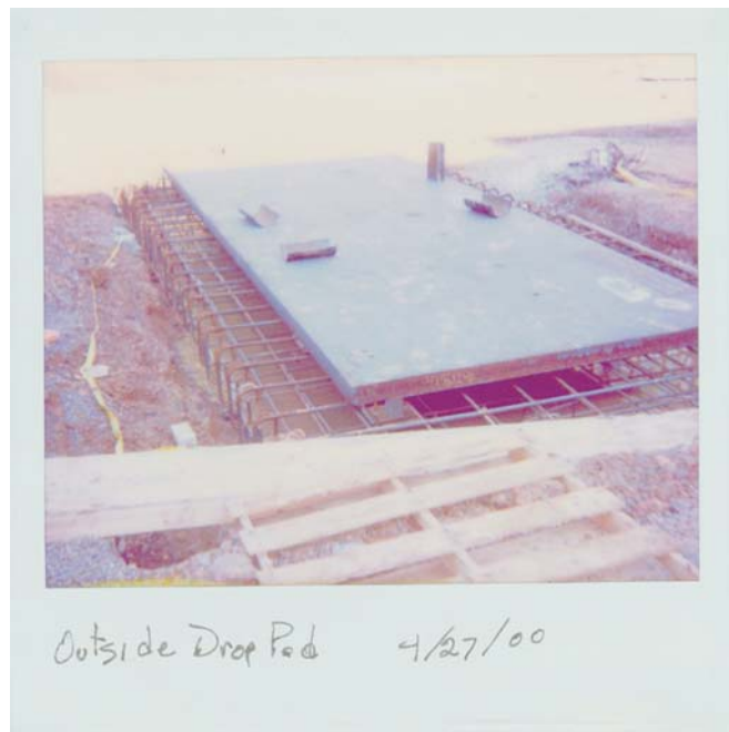
Fig. 7. End view of exterior drop pad during construction.
