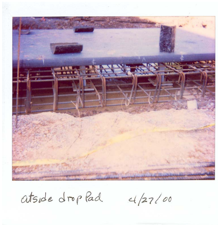
Fig. 6. Side view of exterior drop pad during construction.
