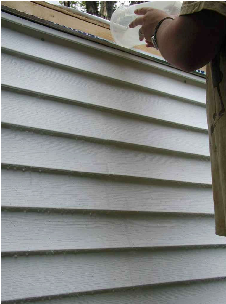
Fig. 11. Water poured behind vinyl at top can be seen emerging and draining on outer face.
