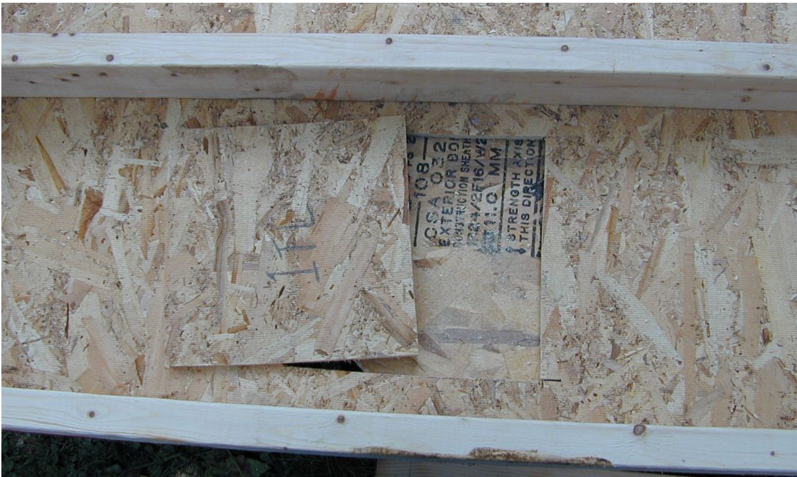
Fig. 5. Exterior sheathing with designed visual openings.
