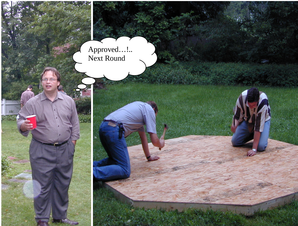
Fig. 4. Approval/certification of the octagon test hut base.
