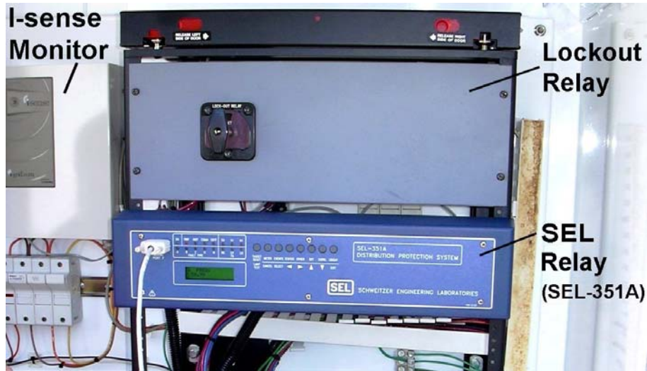
Fig. 2.7. SEL relay and lockout relay in cabinet adjacent to the Service B transformer.
