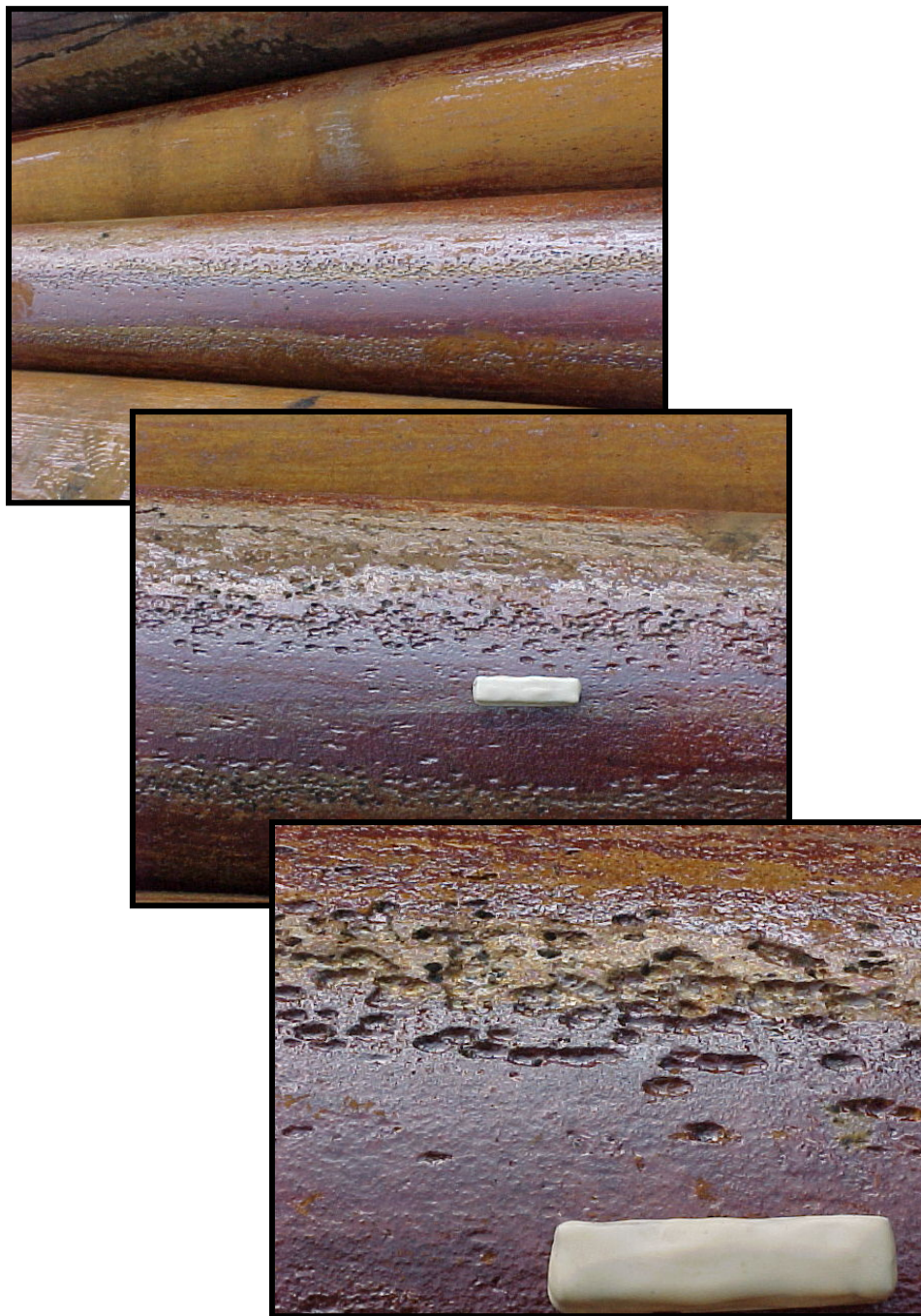
Fig. 3. Three views of a small diameter section of center pipe removed from the digester in June 2003. Note the parallel rows of pits separated by relatively smooth areas. Pits here are generally 40 mils deep and slightly elongated in the longitudinal direction rather than being hemispherical. The white scale marker is 3.5 cm long.
