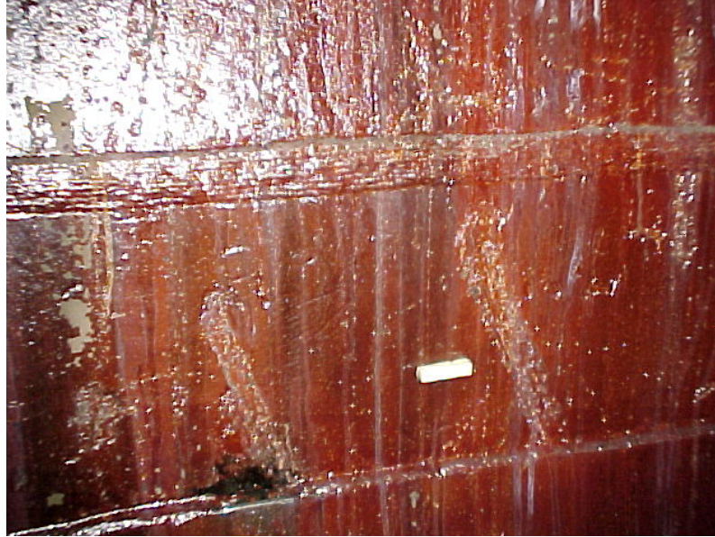
Fig. 6. Transition piece (ring 17) and the round seam weld H18 at the June 2003 inspection. Localized corrosion at this location was not previously documented. Pits near the white scale marker (3.5 cm long) are generally 60-75 mils deep.
