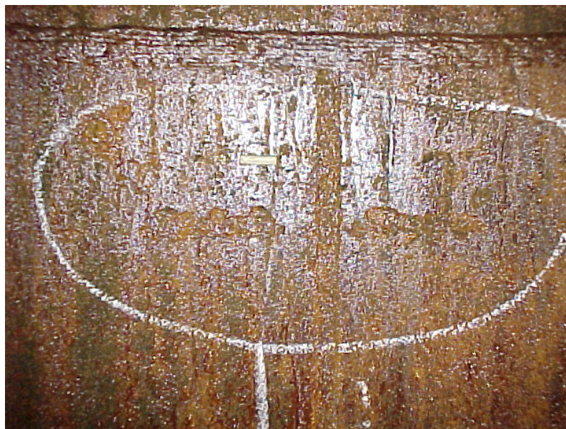
Fig. 8 Views of ring section 12 at the June 2003 inspection. Top: general appearance, showing shallow pits scattered in a mostly unattacked surface. Bottom: some pits appear to have agglomerated in patterns suggesting the location of a former bracket just below the H13 seam weld. White scale marker is 3.5 cm long.
