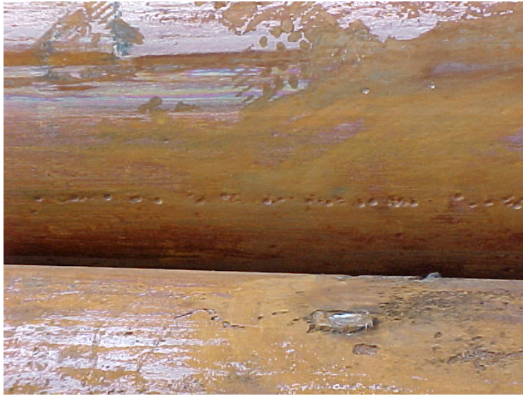
Fig. 4. Large diameter section of the center pipe with a single row of hemispherical pits about 60 mils deep.
