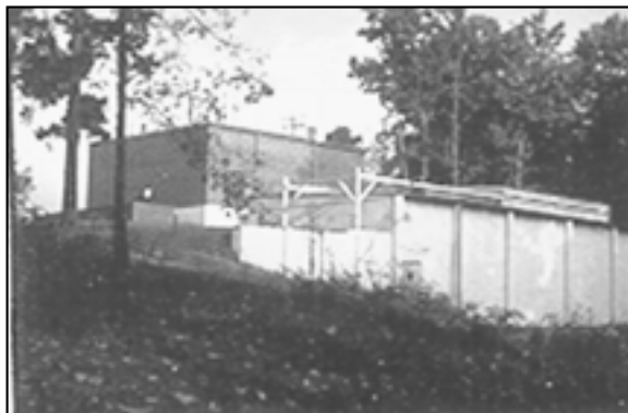
Figure 14. Another Example of a Bunker Storage System.
