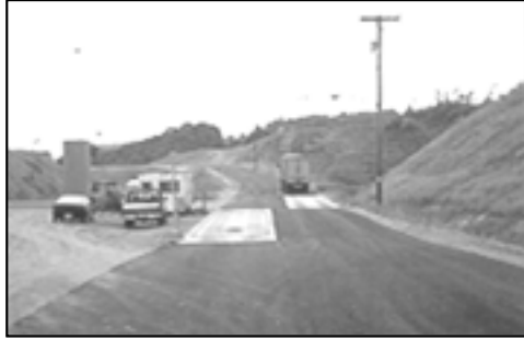
Figure 32. Separate Scales with Bar Code Scanners are Used to Weigh Incoming and Outgoing Trucks at the 90 MW Plant at Hurt, Virginia.
