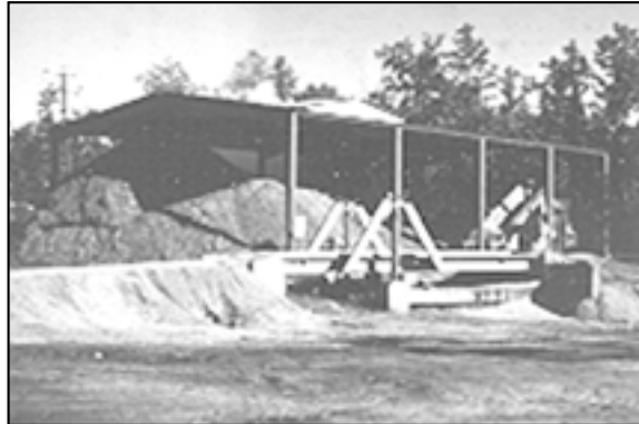
Figure 17. An Open Shed Wood Storage System with a Trailer-Only Dumper in the Foreground.
