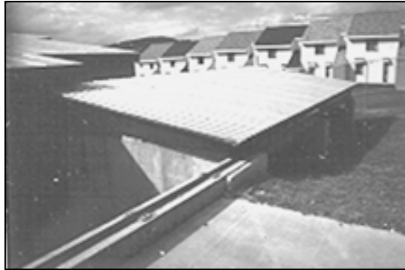
Figure 13. A Bunker Storage System with Roof Retracted to Allow Fuel to be Dumped into Storage.
